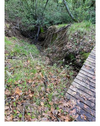
This is the area below the still intact footbridge. Notice the undercutting erosion of the bank. Picture taken on Harms/Damery land looking downhill. This continues to get worse with increased water drainage
