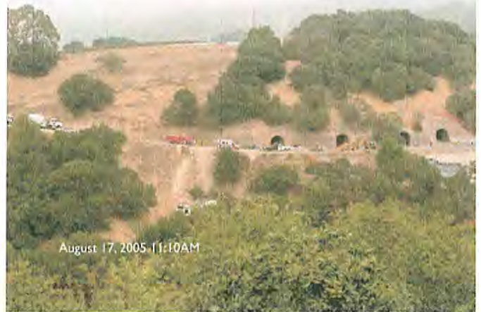
The day a fully-loaded concrete truck tumbled a hundred feet down the canyon wall in 2005.
