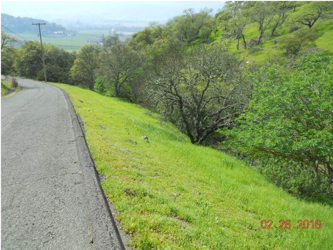
Figure 5. View of section that will be widened approximately two feet along the ruderal verge above the unnamed ephemeral drainage. No vegetation will be removed.
