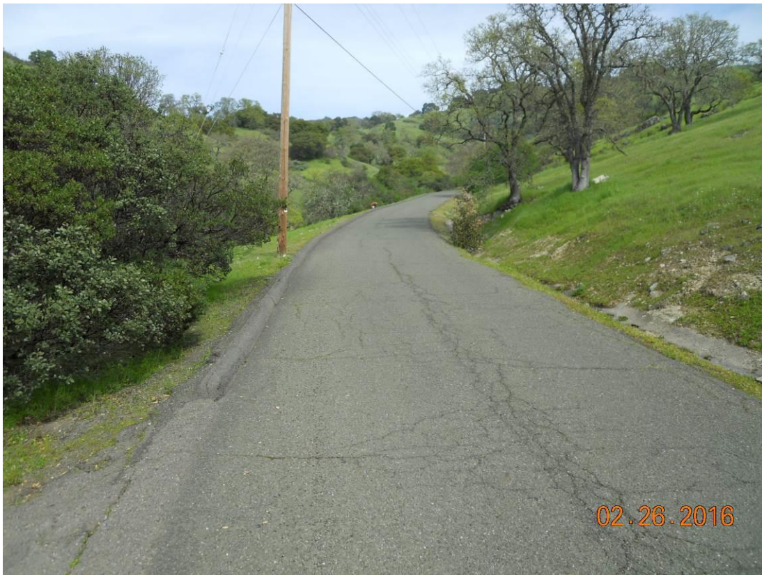
Figure 3. Road section adjacent to the unnamed ephemeral drainage. Widening will occur along the left side and on the upslope side.
