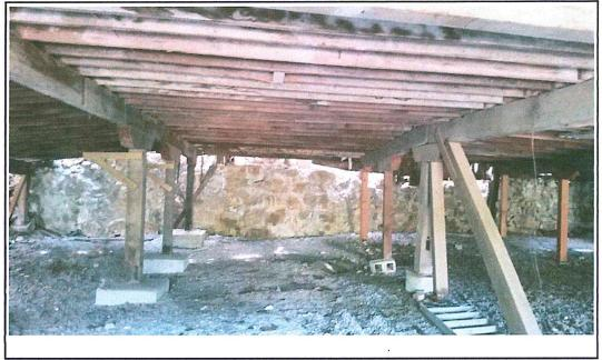
Figure 7. Interior showing failed stone retaining wall at lower level.
