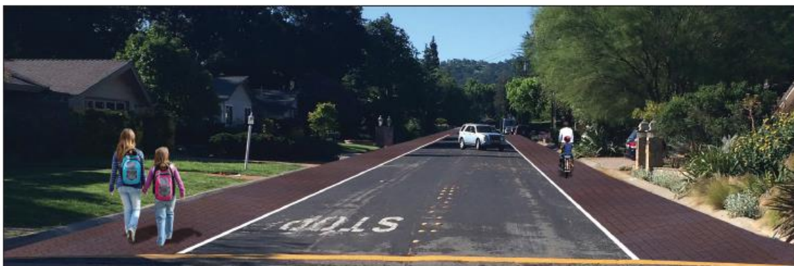
Edgelines and stamped, colored asphalt added
