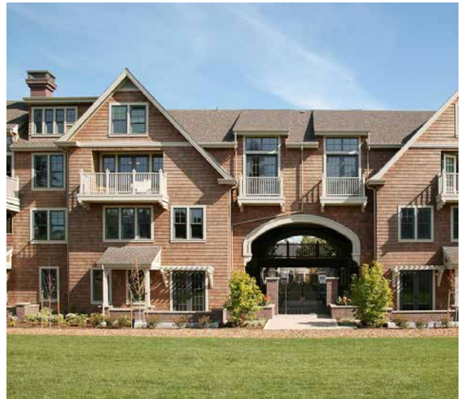
Apartments facing Heritage Park
