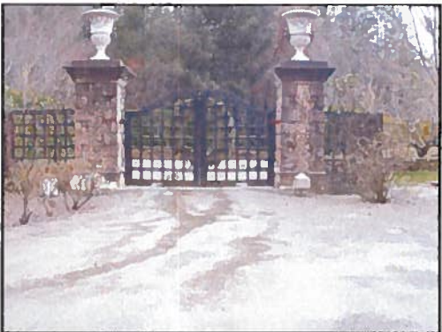
Photo 3: Existing driveway with gated entrance.
