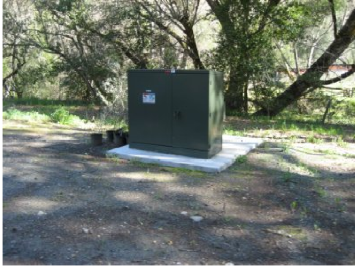
Photo 9: Pad mounted transformer at hammerhead.
