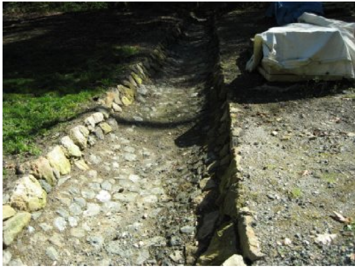
Photo 2: Drainage ditch, lined with rock.
