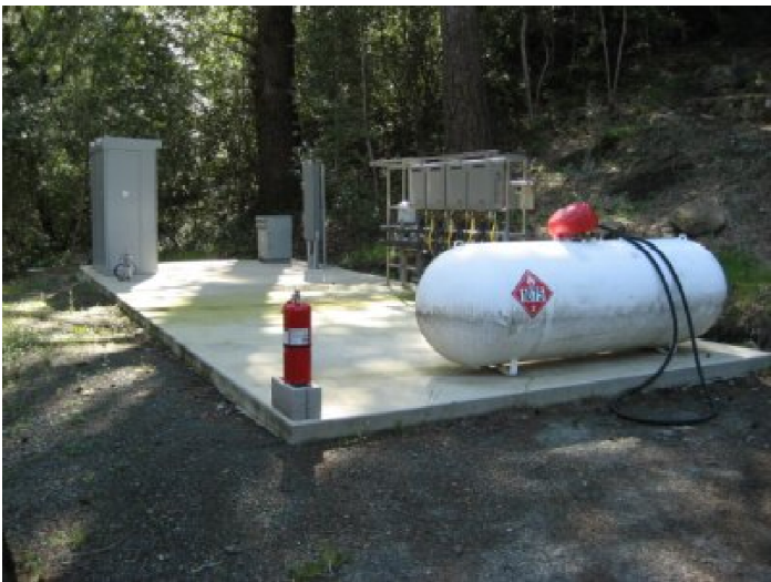
Photo 6: Propane tank, water heaters on concrete pad.
