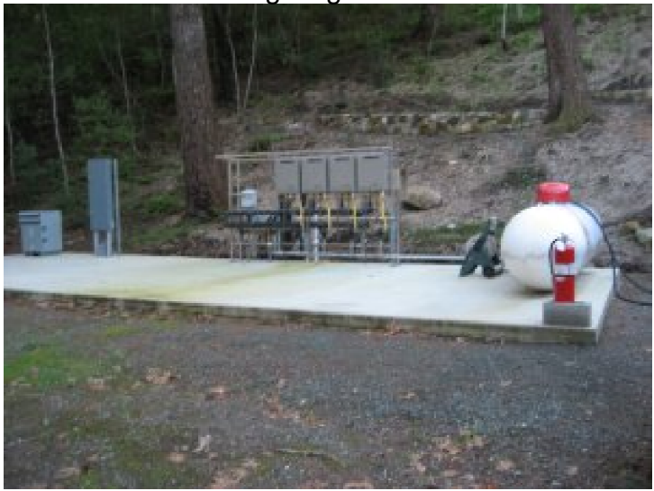
Photo 6: Propane tank, water heaters on concrete pad.
