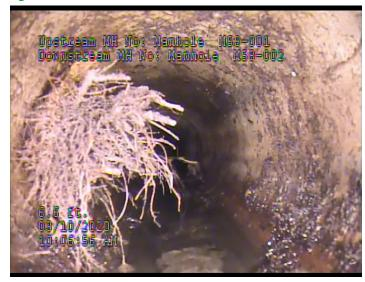
Heavy root intrusion through cracked pipe
