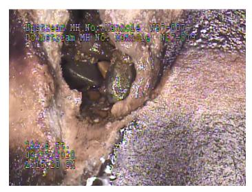
Hole in pipe adjacent to lateral connection
