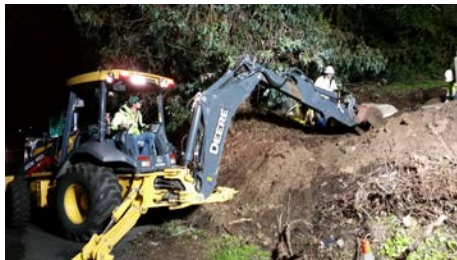
Sewer repair on Silverado Trail
