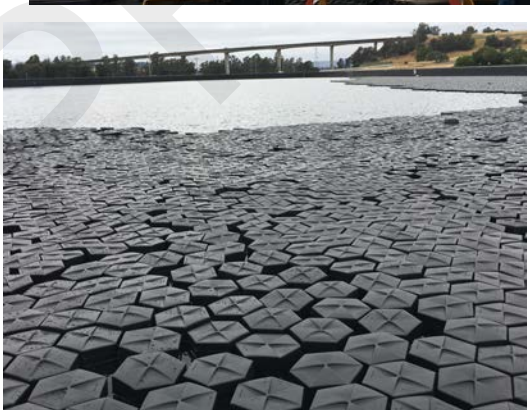
Installation of the floating covers on the recycled water reservoir at the Soscol Water Recycling Facility.
