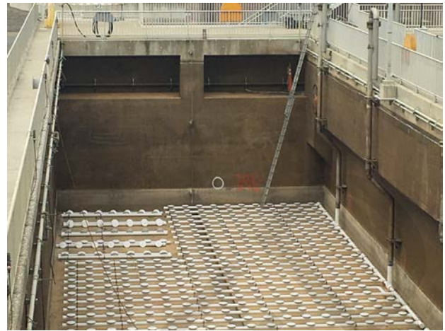
The aeration basin panels were replaced in 2017.
