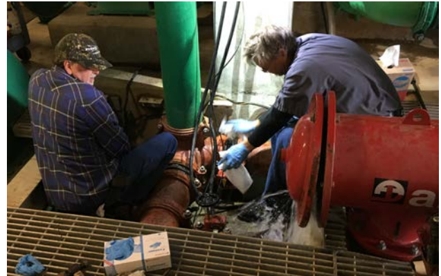
Maintenance technicians installing a valve to the “3-Water” filter.
