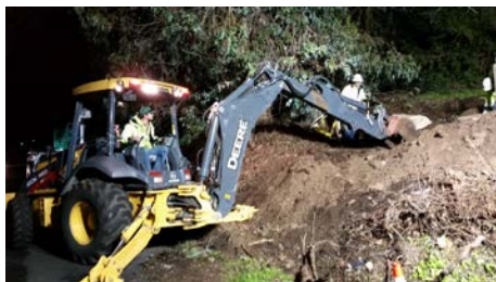
Sewer repair on Silverado Trail
