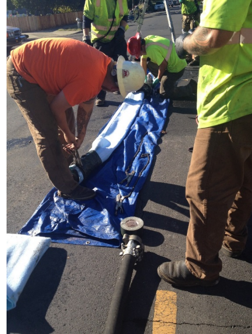
Cured-in-place pipe (CIPP)
