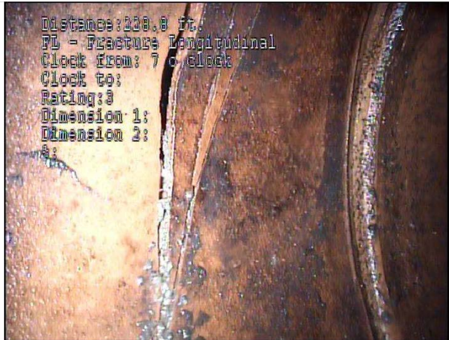
VCP with cracks/fractures
