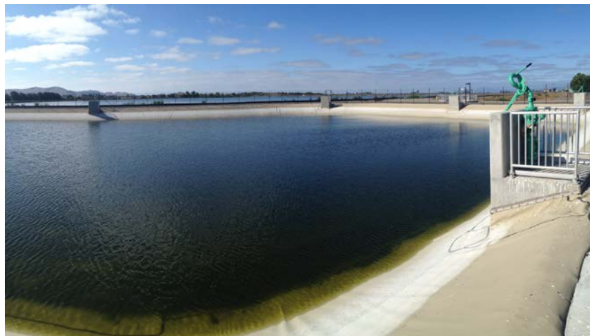
Completed secondary effluent equalization basin
