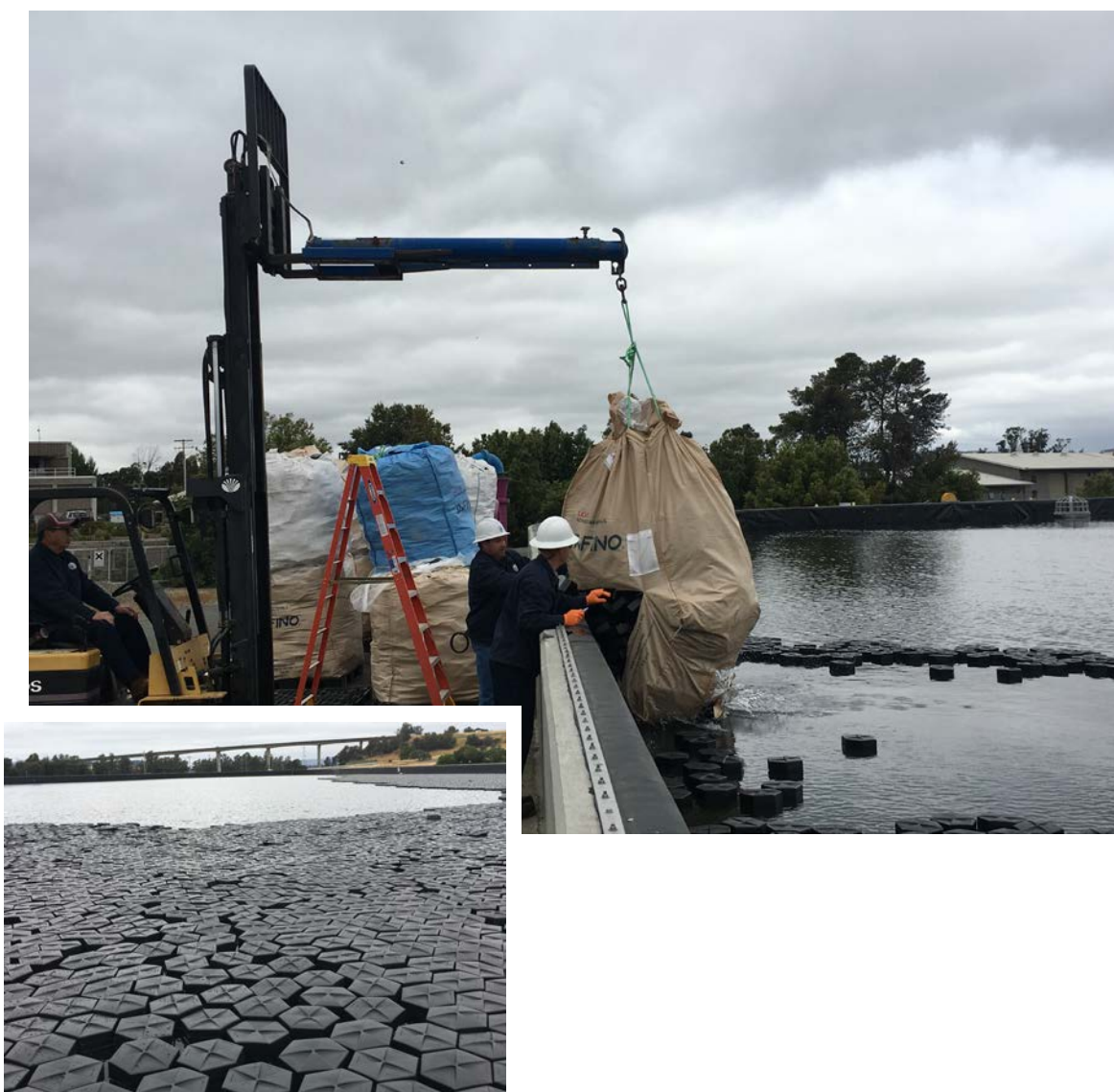
Installation of the floating covers on the recycled water reservoir at the Soscol Water Recycling Facility.
