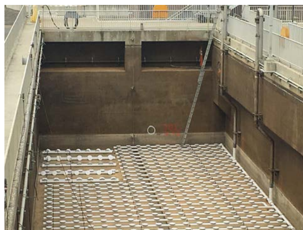
The aeration basin panels were replaced in 2017.
