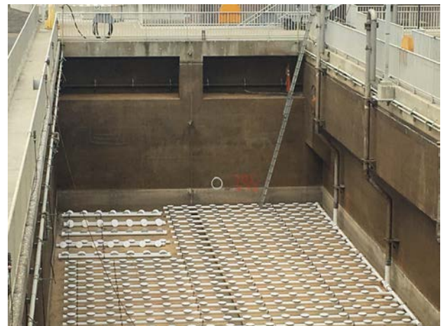
The aeration basin panels were replaced in 2017.
