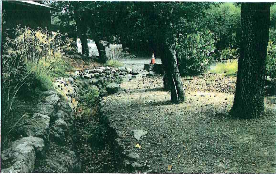
Photograph 5: Unnamed drainage illustrating river-rock creek banks
