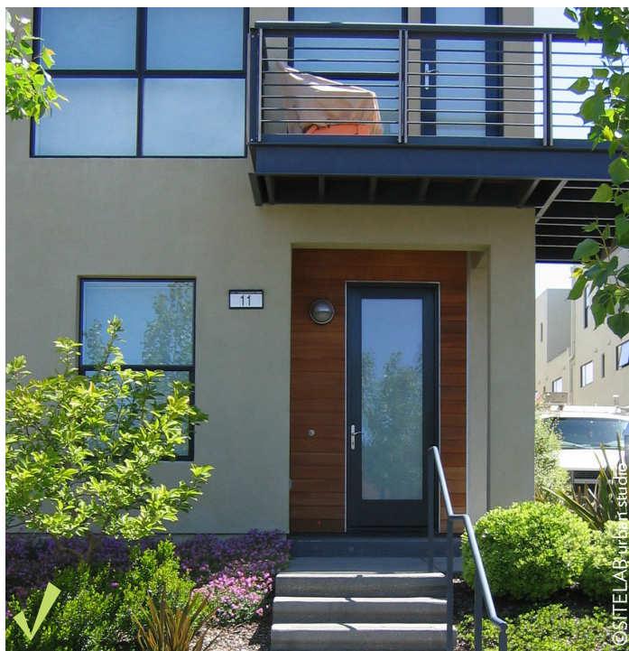
Figure 4.1.6k Exterior Doors. Exterior doors are wood, glass, and steel. Recessed entries with greater height and finished with unique materials distinct from the predominant façade material.
