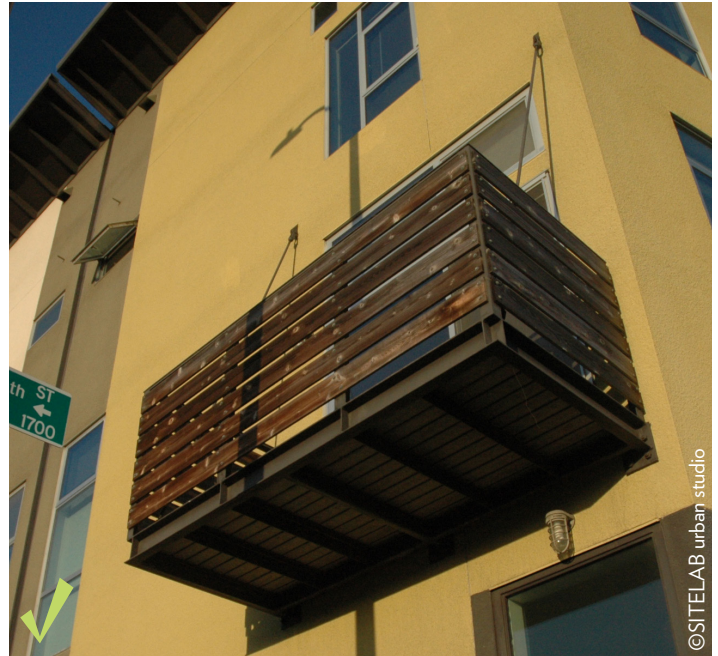
Figure 4.1.4j Well-detailed steel and wood hanging balconies with substantial materials and attention to the method of joinery.
