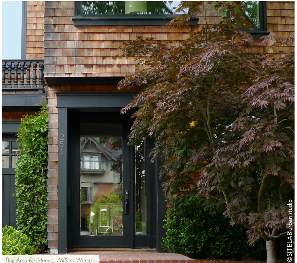
Figure B.2.1h Recessed entry framed with dark timber creates a clear hierarchy of materials between the overall shingle and the dark details and accents. Material changes correspond to openings, entries, and projections.
