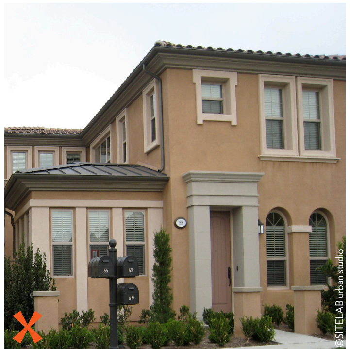
Figure 4.1.6p Roofline and Eaves. Good (above): Eave depth adds variety and articulates the façade. Good (bottom left): Flat roof has horizontal articulation with eave and reveal. Bad (bottom right): Minimal cornice depth does not meet minimum eave depth and no separation from windows creates unbalanced composition.
