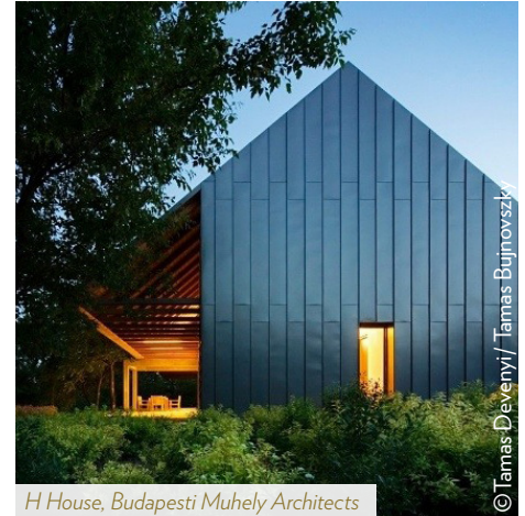
Figure B.3.1b Gable-roof forms with emphasis on planes and surfaces. Forms refer to simple functionality of farm structures. Materials provide texture and ornamentation. Corrugated and panelized metal are industrial and contemporary.
