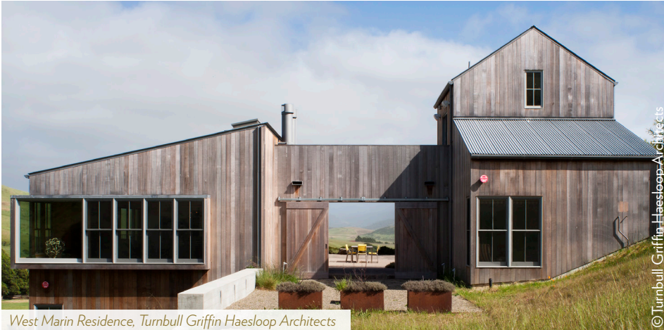
Figure B.3.1b Gable-roof forms with emphasis on planes and surfaces. Forms refer to simple functionality of farm structures. Materials provide texture and ornamentation. Corrugated and panelized metal are industrial and contemporary.
