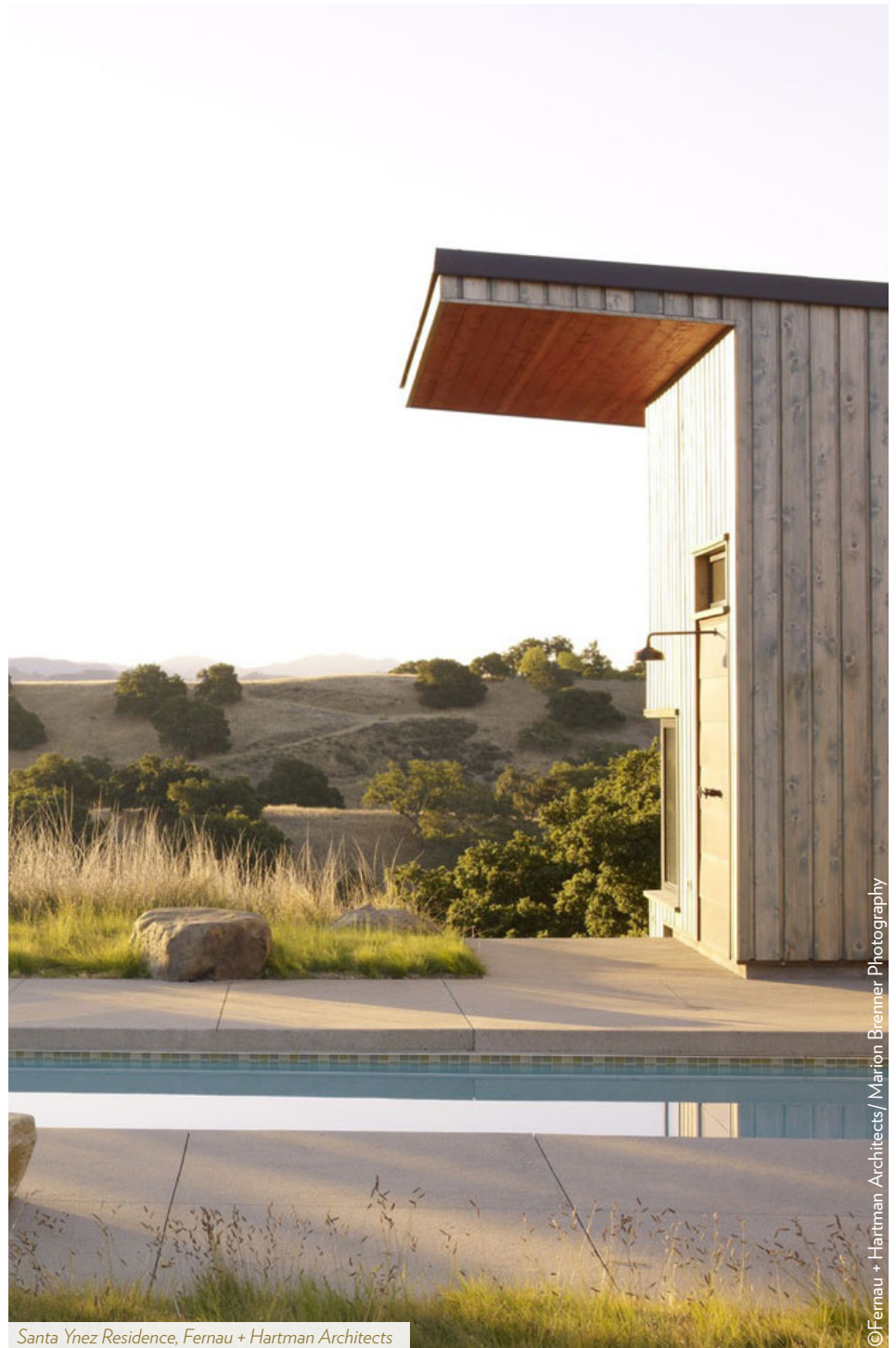
Figure B.3.1a Vertical clapboard with regional materials connects to farm vernacular. This is combined with the contemporary components of the canted, asymmetrical roof and the deep eave.
