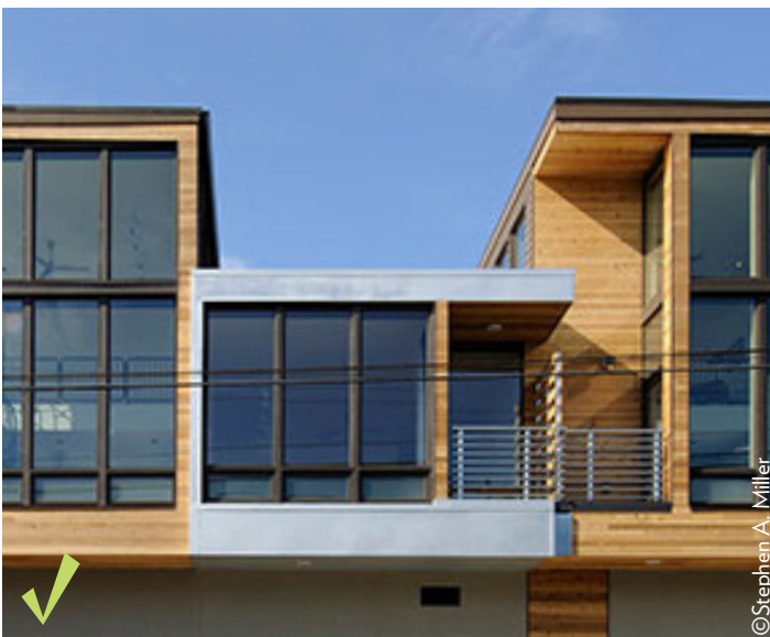
Figure 4.1.6o Roof Articulation. Good (left): Roof articulation reflects interior spaces and expresses massing. Bad (right): Single continuous roofline does not modulate or address façade projections.
