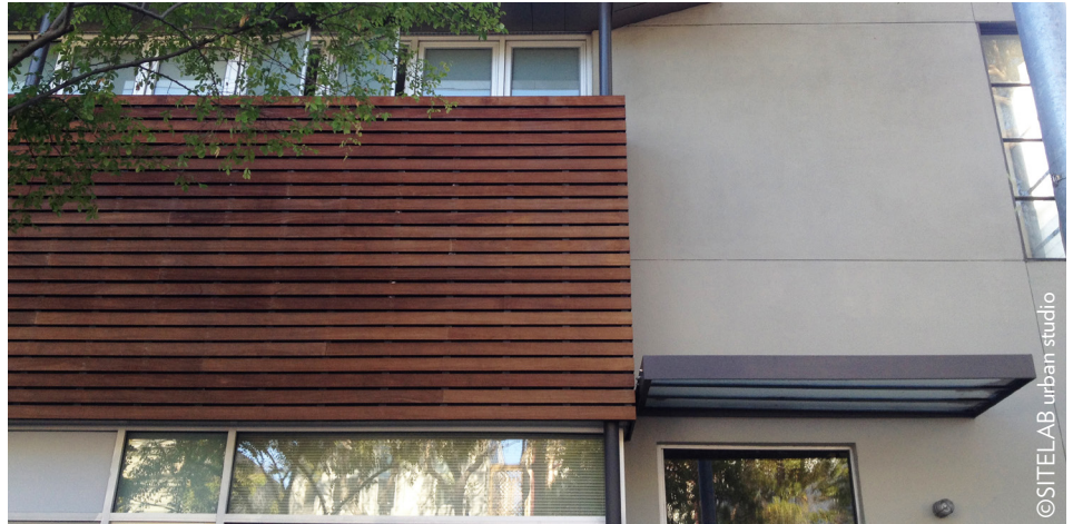
Figure B.2.1e Slatted wood projection adds a layered horizontal texture to the smooth and basic stucco volume.
