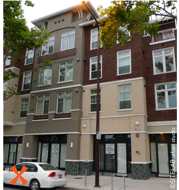
Figure 4.1.3e Material and Façade Composition. Good (left): Clear material palette is associated with façade projections in a balanced composition. Bad (right): Multiple façade materials are not coordinated with projections and change at three different levels.
