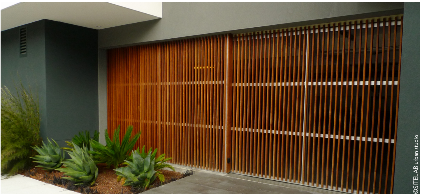
Figure 4.7.5a Whereas the screened opening to structured parking allows for air flow exchange, the drive aisle is narrow to minimize paved area and instead allow for more plantings. Wood slats screen the parking and vehicles from view, allow for air flow, and provide visual interest with quality materials.
