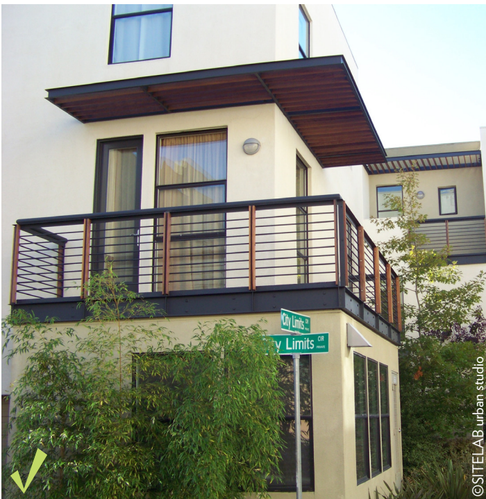
Figure 4.1.4k Balconies and Decks (left) Well-detailed balcony integrated with massing transition, partial awning, and wrapping the corner. (right) Well-detailed open deck with slatted wood shading system and attention to the method of joinery.
