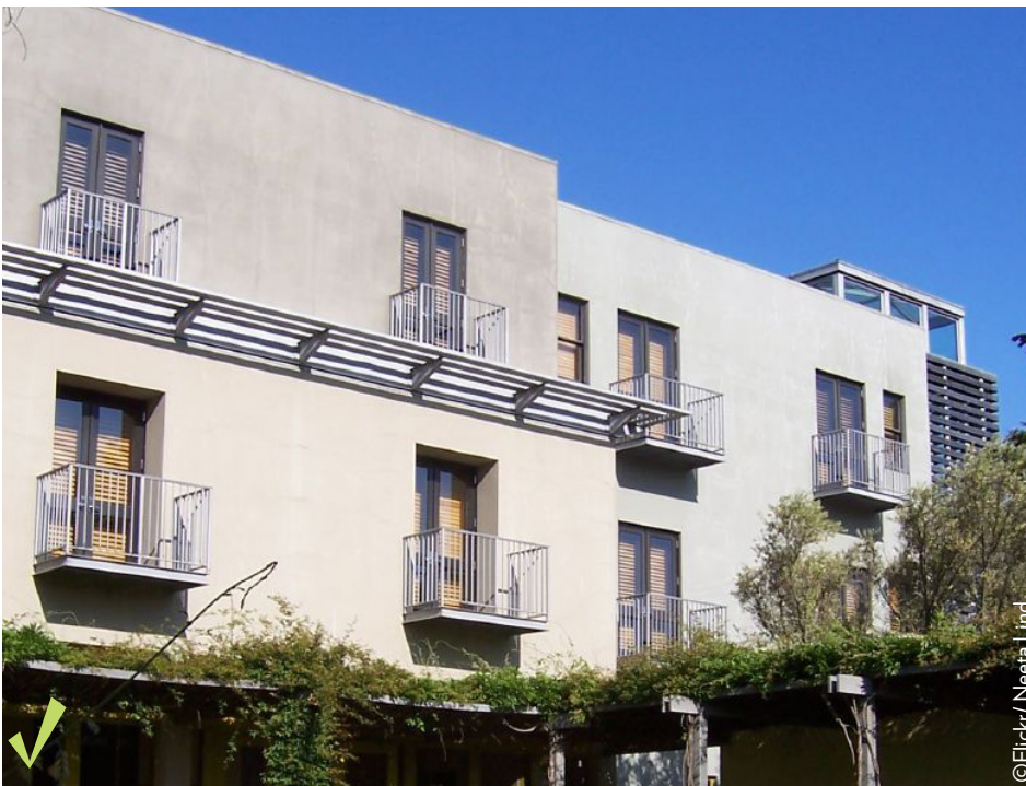
Figure 4.2.6d Good (left): Recessed windows create perceivable wall thickness. Bad (right): Flush window and thin framing yields no shadow and a flat façade.
