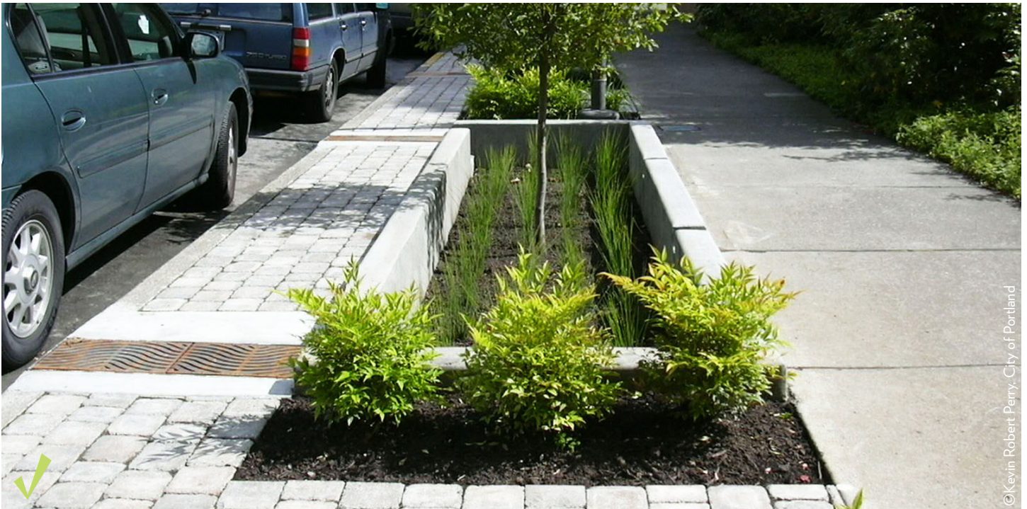
Figure 4.8.1a An urban rain garden is a sustainable streetscape treatment. Runoff flows from the street through the curb cut channels into the rain garden planter, slowing flow of runoff into the stormsewer, allowing for infiltration, and irrigating vegetation.
