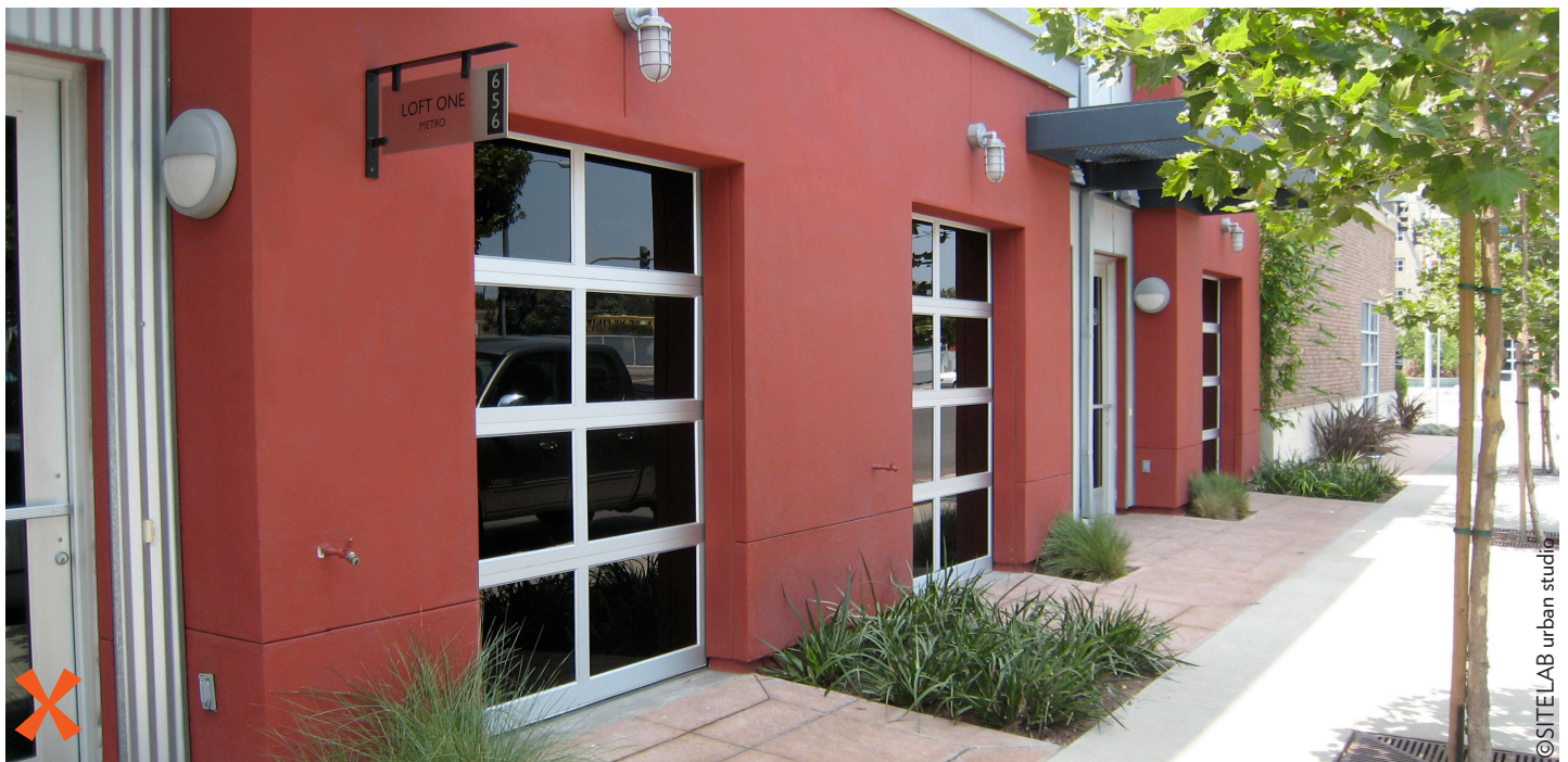
Figure 4.2.6e Doors. Good (top left and right): Exterior doors are wood, glass, and steel with transparency; They have recessed entries and are finished with unique materials. Bad (bottom): Dark glazing prohibits transparency from adjacent sidewalk, reducing active street frontage.
