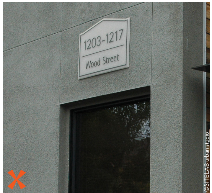
Figure 4.1.6s Numbering. Good (left): Address number is small and coordinated with materials. Bad (Right): Address numbers are large and part of a larger address sign.
