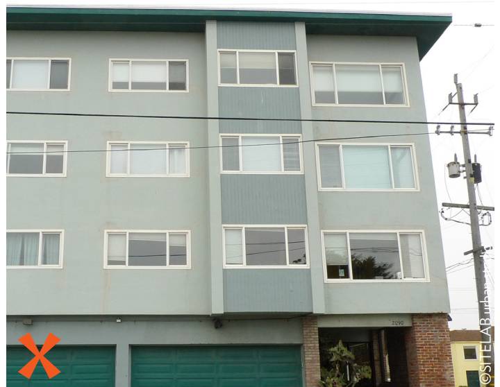
Figure 4.1.6o Roof Articulation. Good (left): Roof articulation reflects interior spaces and expresses massing. Bad (right): Single continuous roofline does not modulate or address façade projections.
