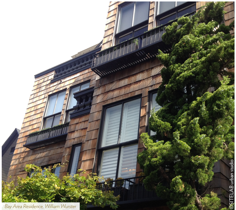
Figure B.2.1c Shingle façade creates building texture and patterning integral to the material. There is a clear hierarchy of local materials among the shingles, metal detailing for projections, and black window reveals.
