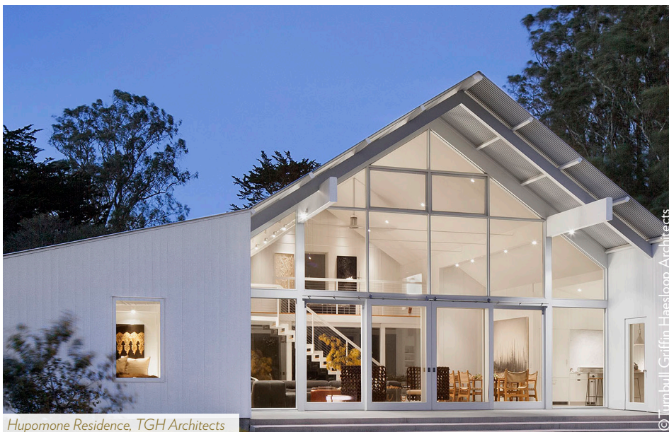
Figure B.3.1j Interior structure and space of simple, gable-roofed form is revealed by recessed, floor-to-gable glass curtain wall.
