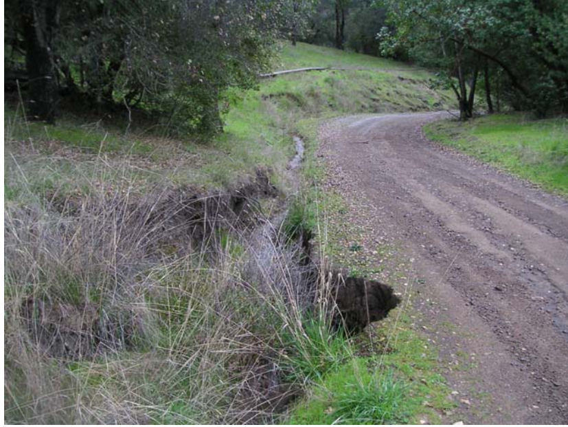
Figure 6. Rills and Gullies on a Compacted Dirt Road
