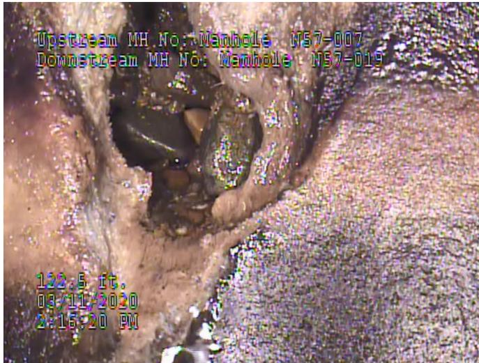
Hole in pipe adjacent to lateral connection
