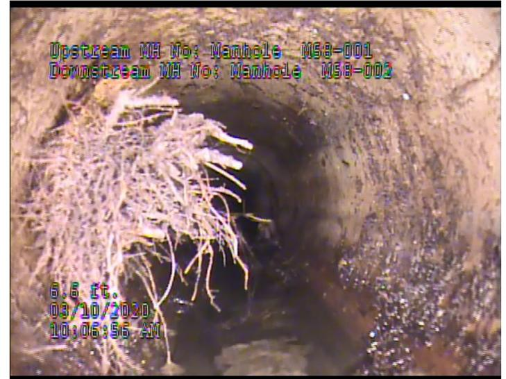
Heavy root intrusion through cracked pipe
