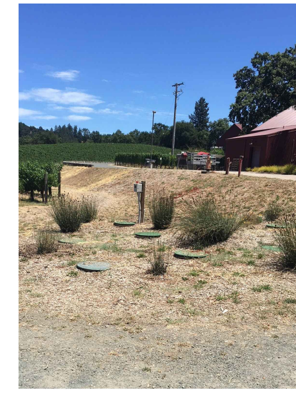
PHOTOGRAPH 7 EASTERLY VIEW OF THE WASTEWATER TANK LIDS
