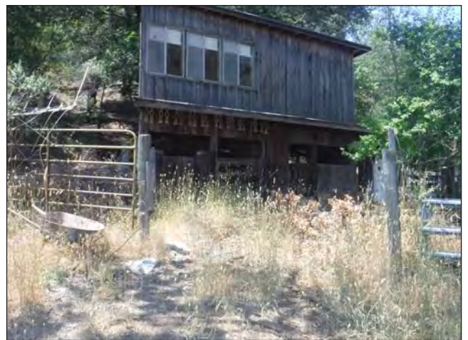
PHOTO 4: Southwest building of Home Site.
