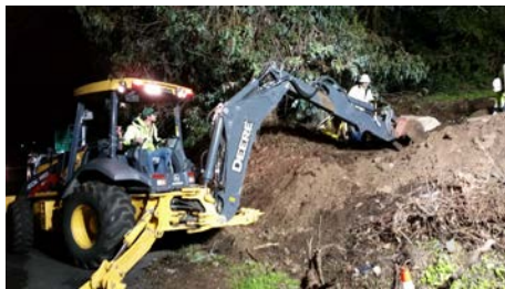
Sewer repair on Silverado Trail
