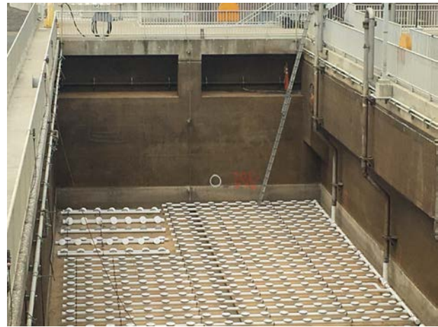
The aeration basin panels were replaced in 2017.
