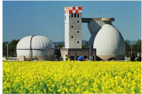
Soscol Water Recycling Facility
