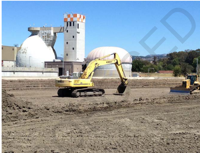
Construction of the secondary effluent equalization basin in 2014
