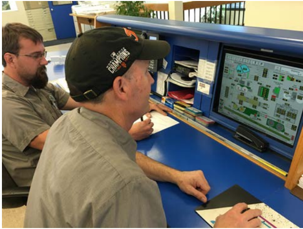
Overseeing plant operations via SCADA interface
