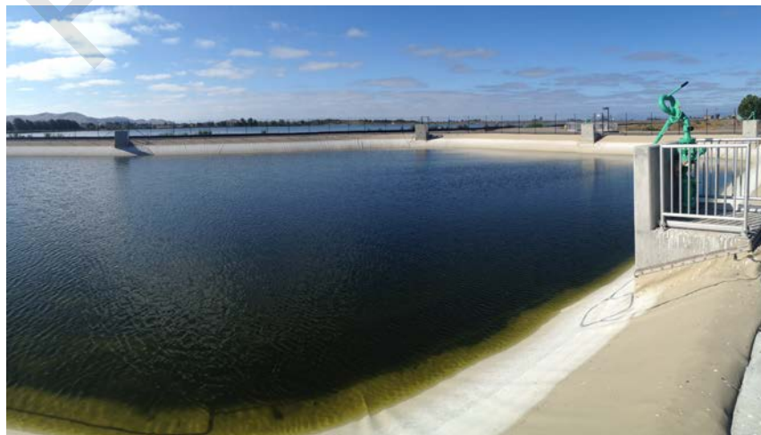
Completed secondary effluent equalization basin
