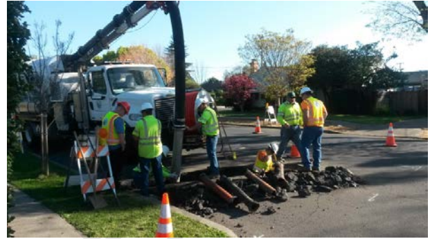
Collection system workers excavate a sewer lateral to make repairs
