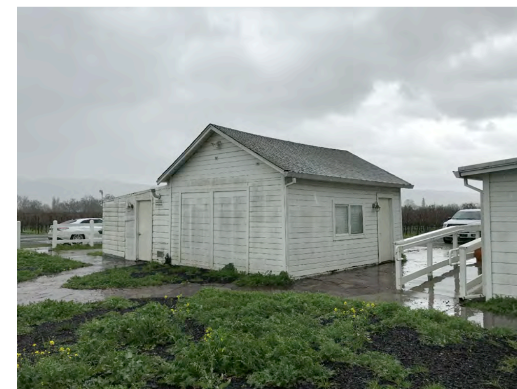
GARAGE: NORTHWEST CORNER
