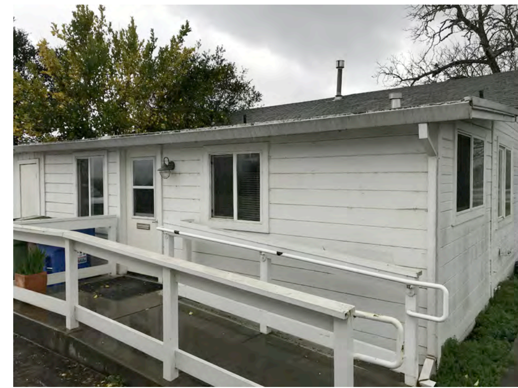
HOUSE: NORTHEAST CORNER
