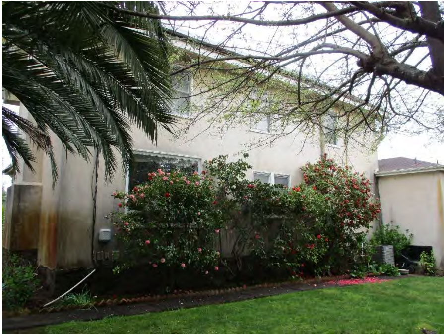
Photo showing the south elevation, facing north/northeast.
