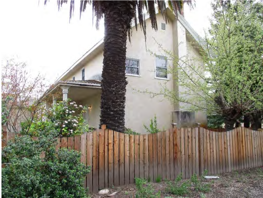
Photo showing the west elevation, facing south/southeast.
