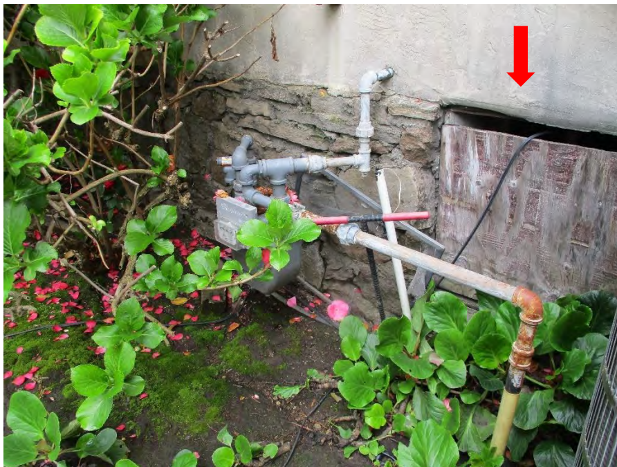
Photo showing the stone foundation, as well the boarded up basement window.
