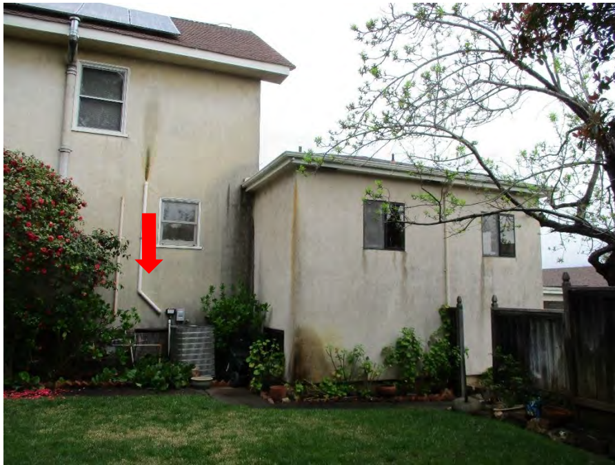
Photo showing the south elevation, facing north/northeast.
