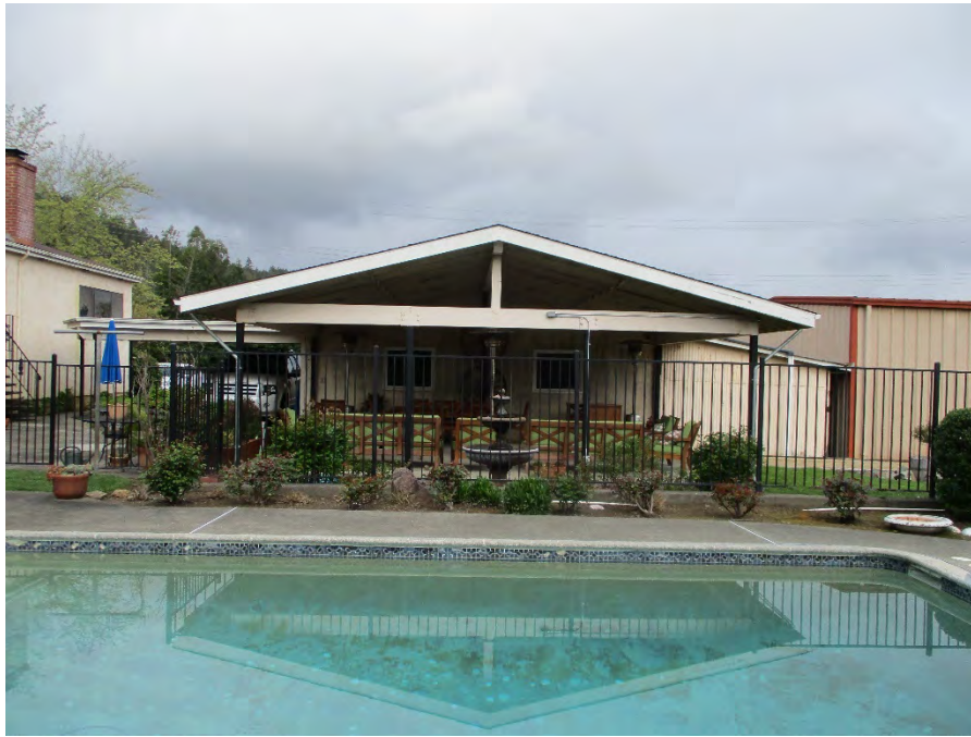
Figure 20. Photo showing the south façade, facing north.
