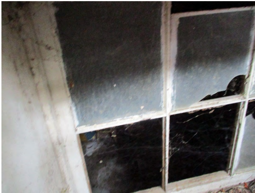
Figure 15. Photo showing the original multi-light basement window along the south elevation.
