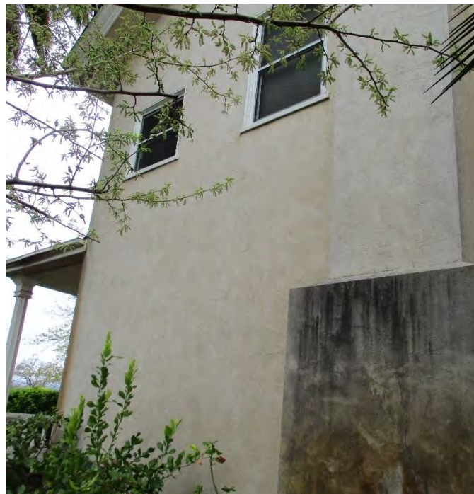
Photo showing the west elevation, facing east.
