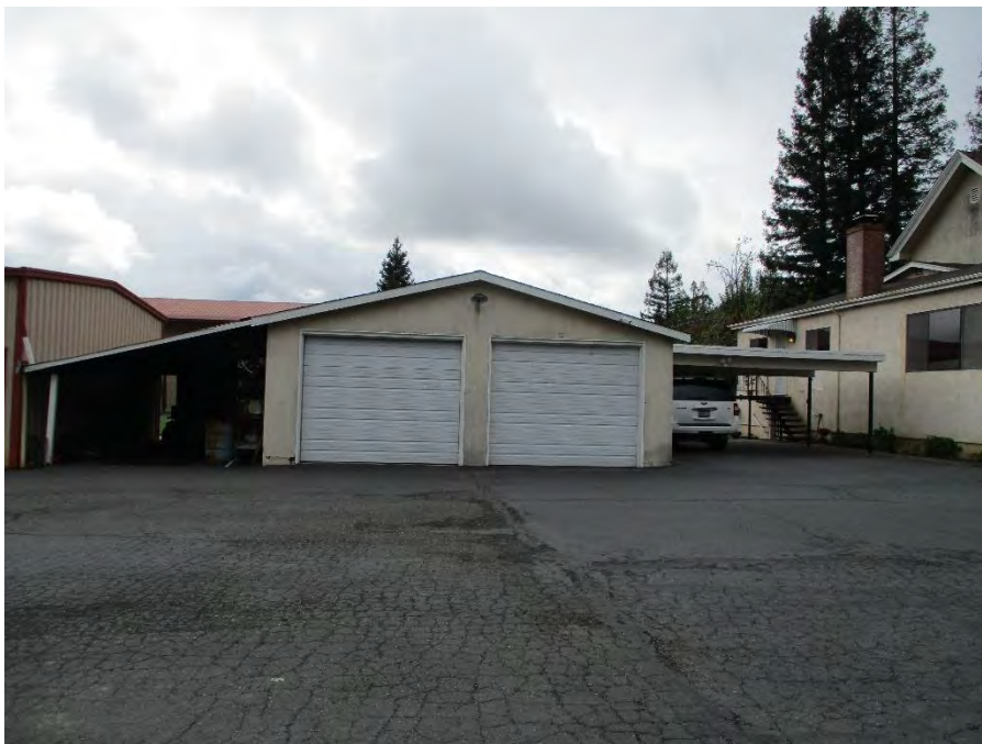
Photo showing the north elevation, facing south.
