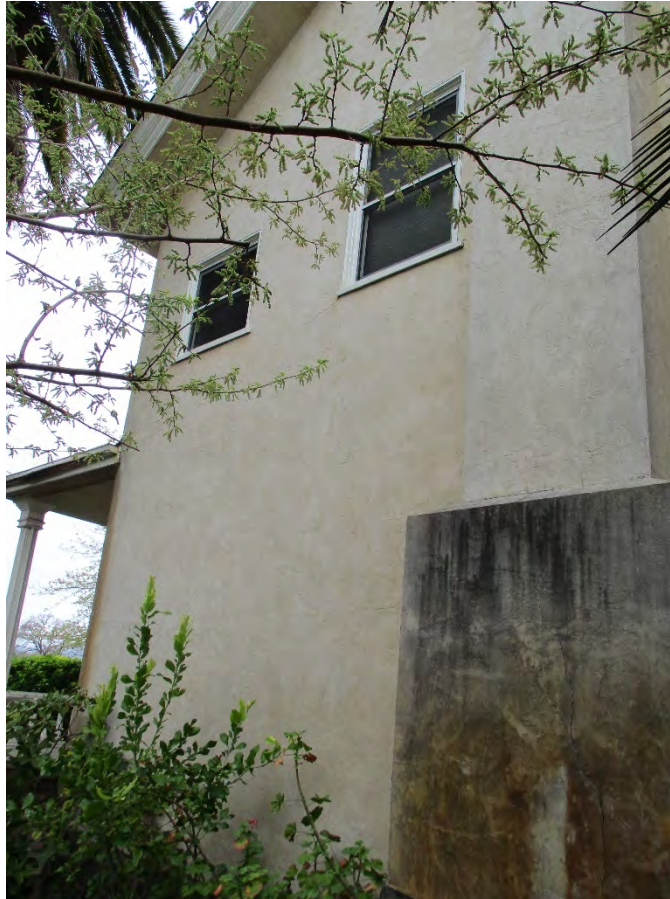
Figure 11. Photo showing the west elevation, facing east.
