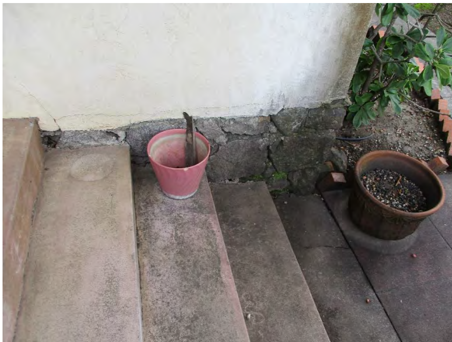
Photo of the foundation of the ca. 1880 house.
