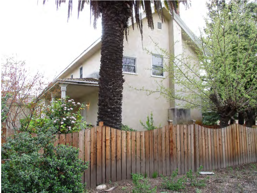
Figure 10. Photo showing the west elevation, facing south/southeast.
