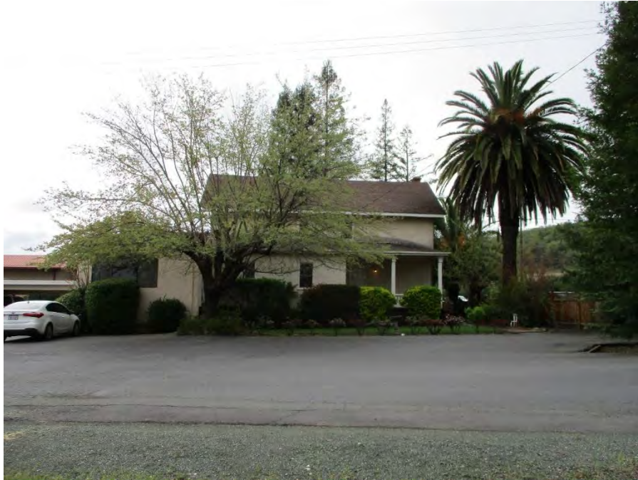
Photo showing north elevation, facing south.
