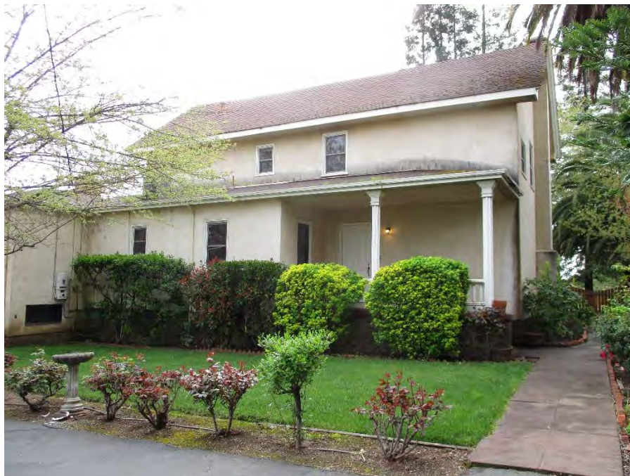
Photo showing north elevation, facing south
