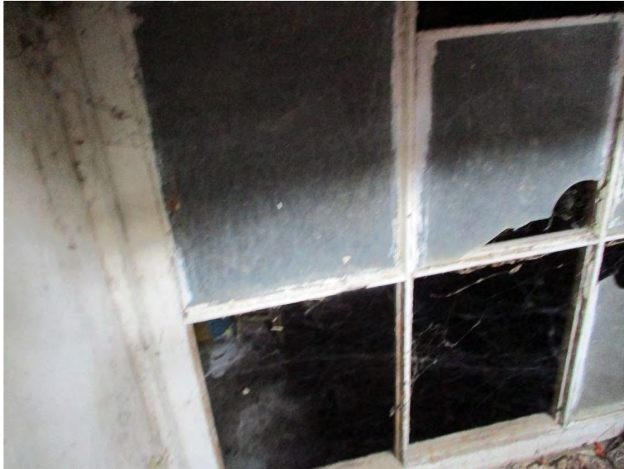
Photo showing the original multi-light basement window along the south elevation.
