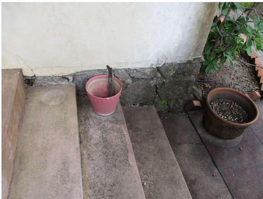
Figure 9. Photo of the foundation of the ca. 1880 house.
