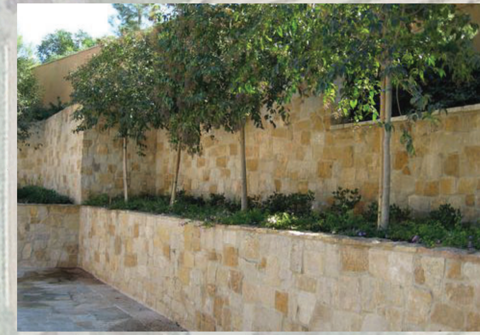
TIERED LANDSCAPE WALLS ALONG ENTRY DRIVE
