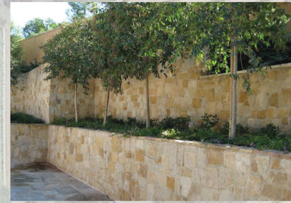
TIERED LANDSCAPE WALLS ALONG ENTRY DRIVE
