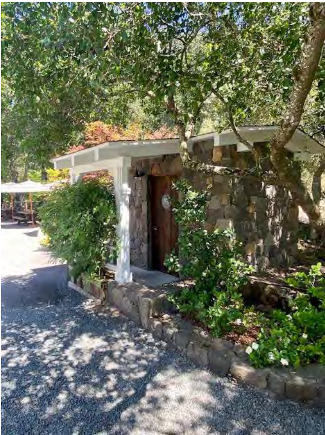
ADA Bathroom – Front:
