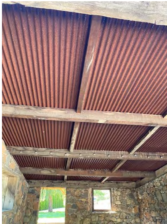
Truck Shelter Roof (corrugated metal):
