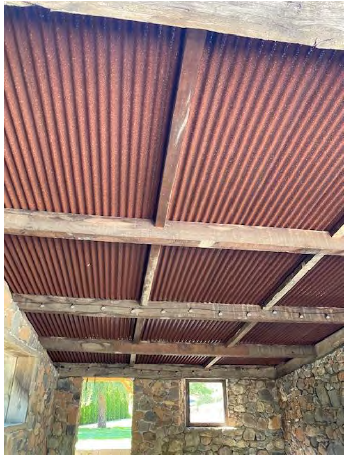
Truck Shelter Roof (corrugated metal):
