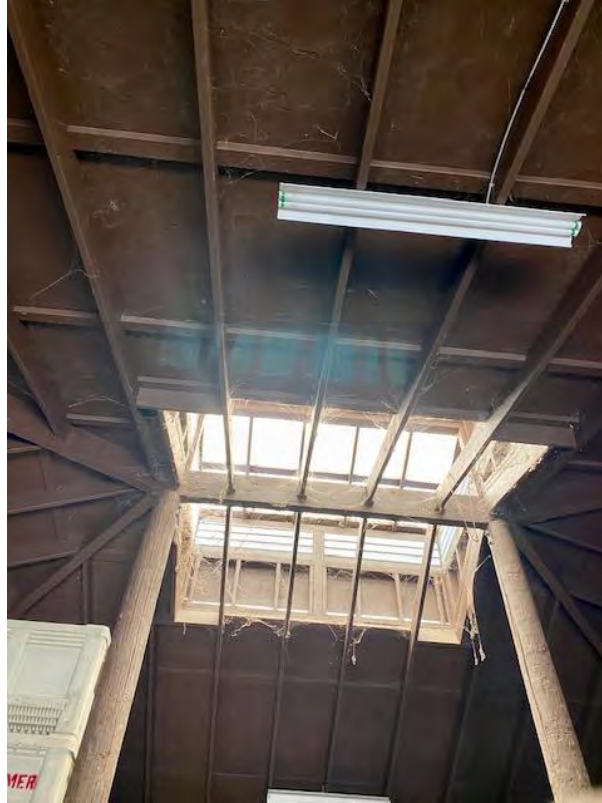
Barn Ceiling Wood:
