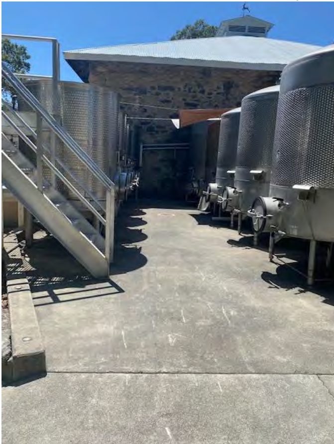
Concrete Pad (Tanks on old concrete pad above Wine Press 15.4'x41' – 635.5 s.f):
