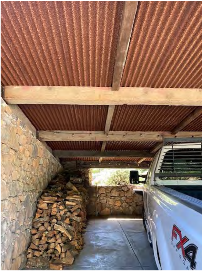
Truck Shelter Roof (corrugated metal):
