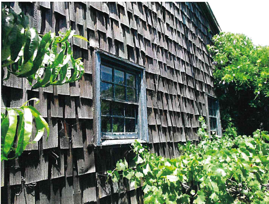
Figure 13. South elevation, showing the two six-over-six double hung wood windows.
