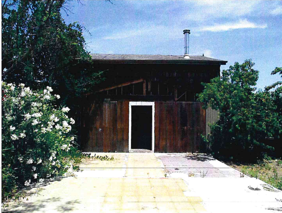
Figure 14. West elevation, facing east.
