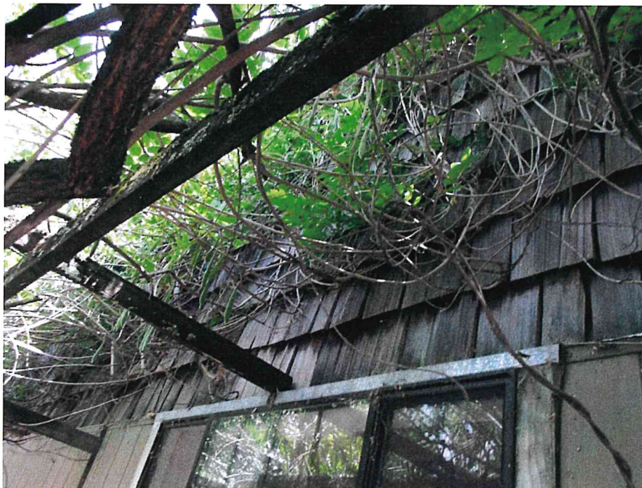
North elevation, showing the modifications to the ca. 1900 barn.
