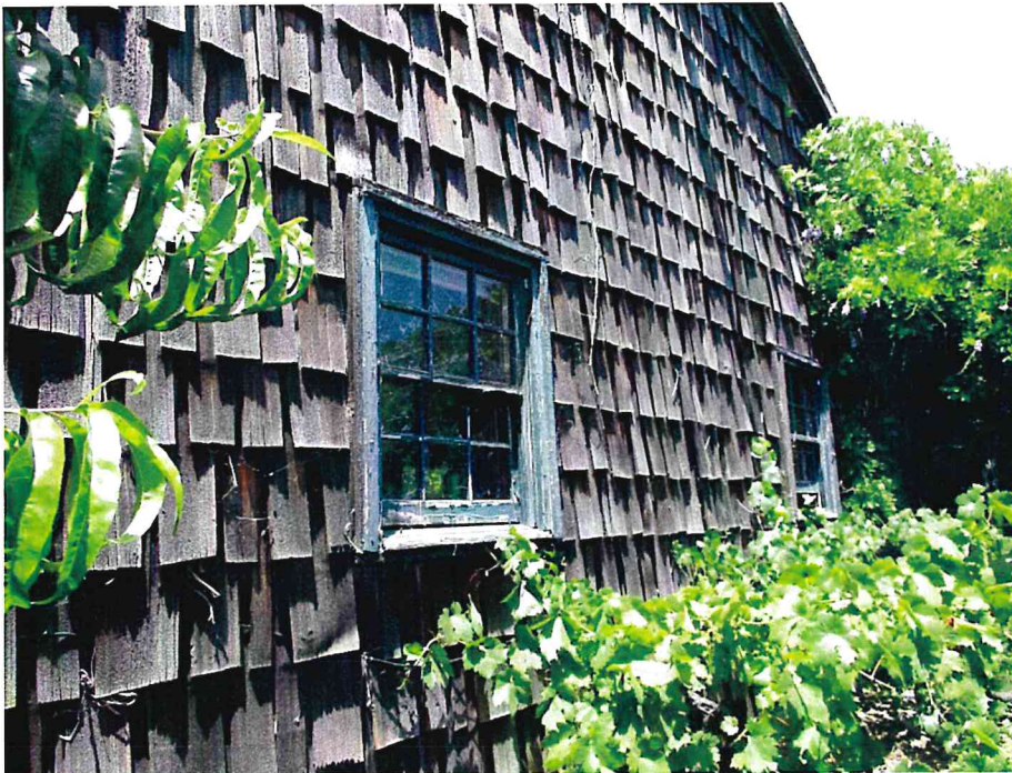
South elevation, showing the two six-over-six double hung wood windows.
