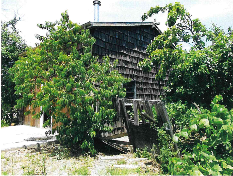
Figure 12. South elevation, facing north, northeast.
