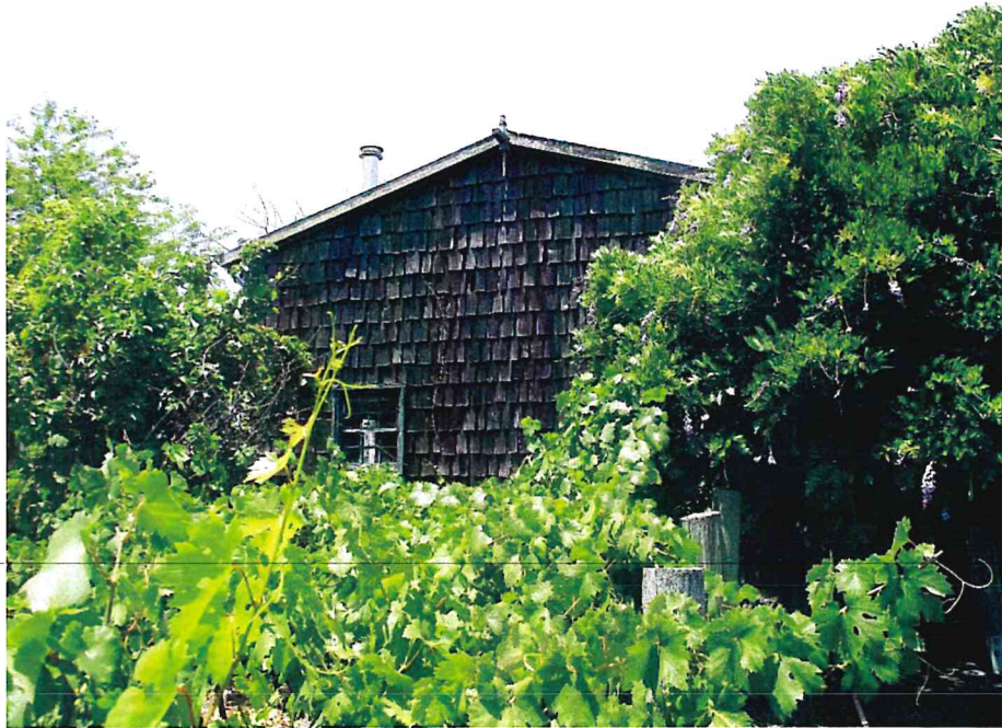
Figure 11. South elevation, facing north.
