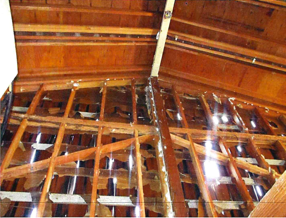
Interior, showing the roof truss and wall system.
