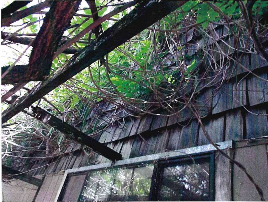
Figure 8. North elevation, showing the modifications to the ca. 1900 barn.
