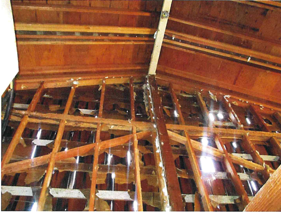
Figure 15. Interior, showing the roof truss and wall system.
