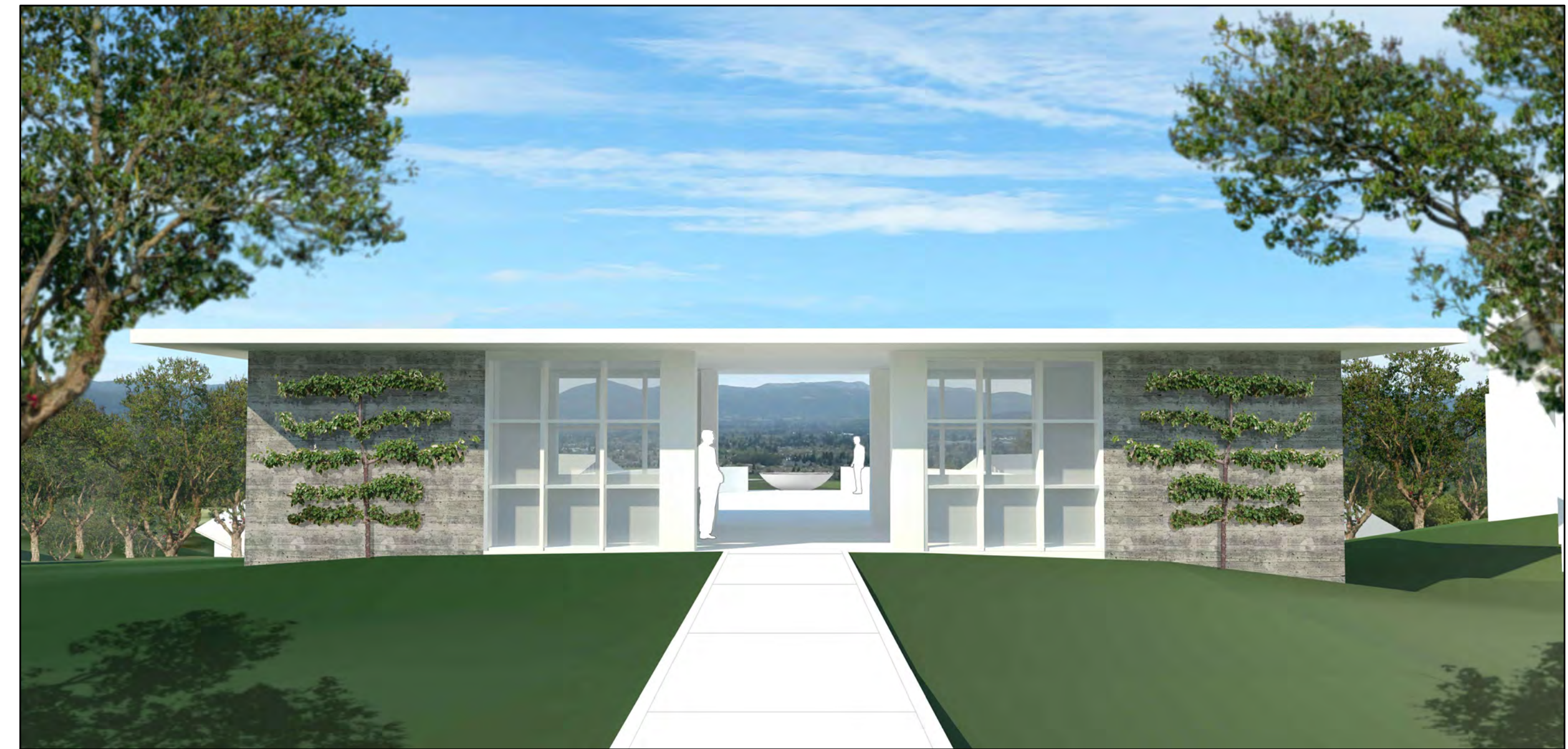
VIEW LOOKING THROUGH ROTUNDA PAVILLION
