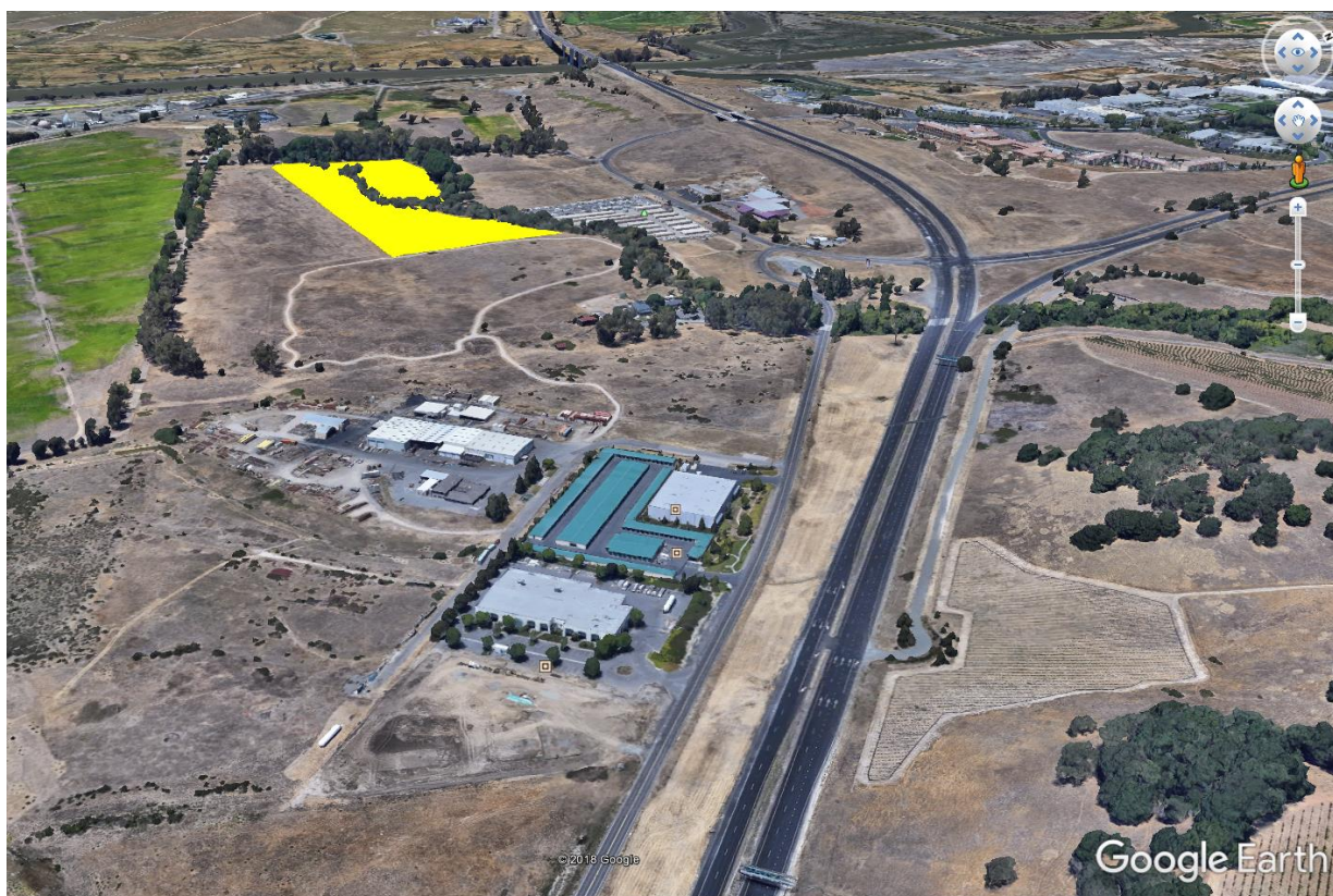
Figure 6. View from Southeast of the Project site from an Elevated Viewpoint across Hwy 12; The Yellow Area is the Project site Footprint within the Perimeter Fence.
