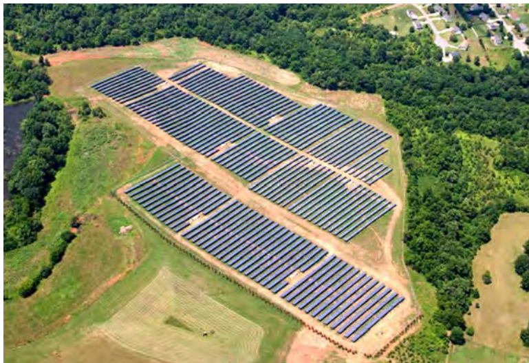
Figure 1: Utility-scale solar facility (5 MW AC ) located in Catawba County. Source: Strata Solar
