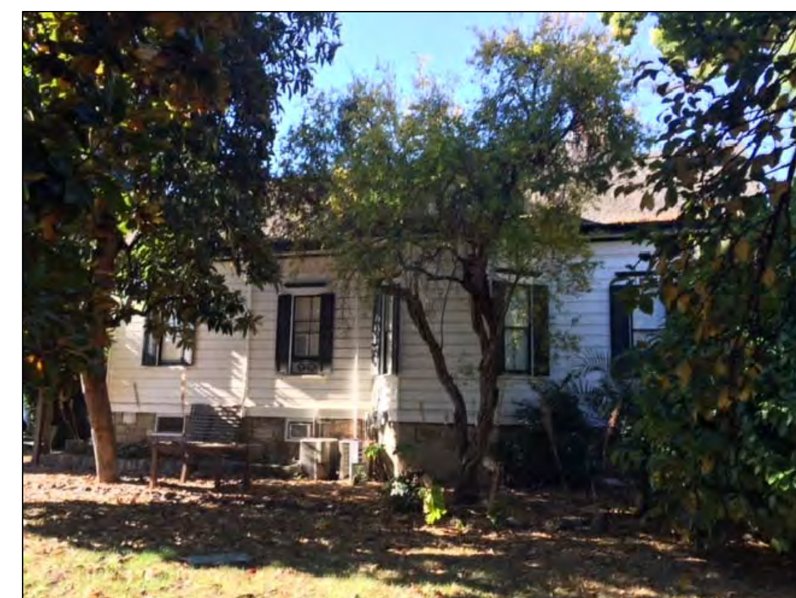
VIEW OF EAST SIDE OF BUILDING
