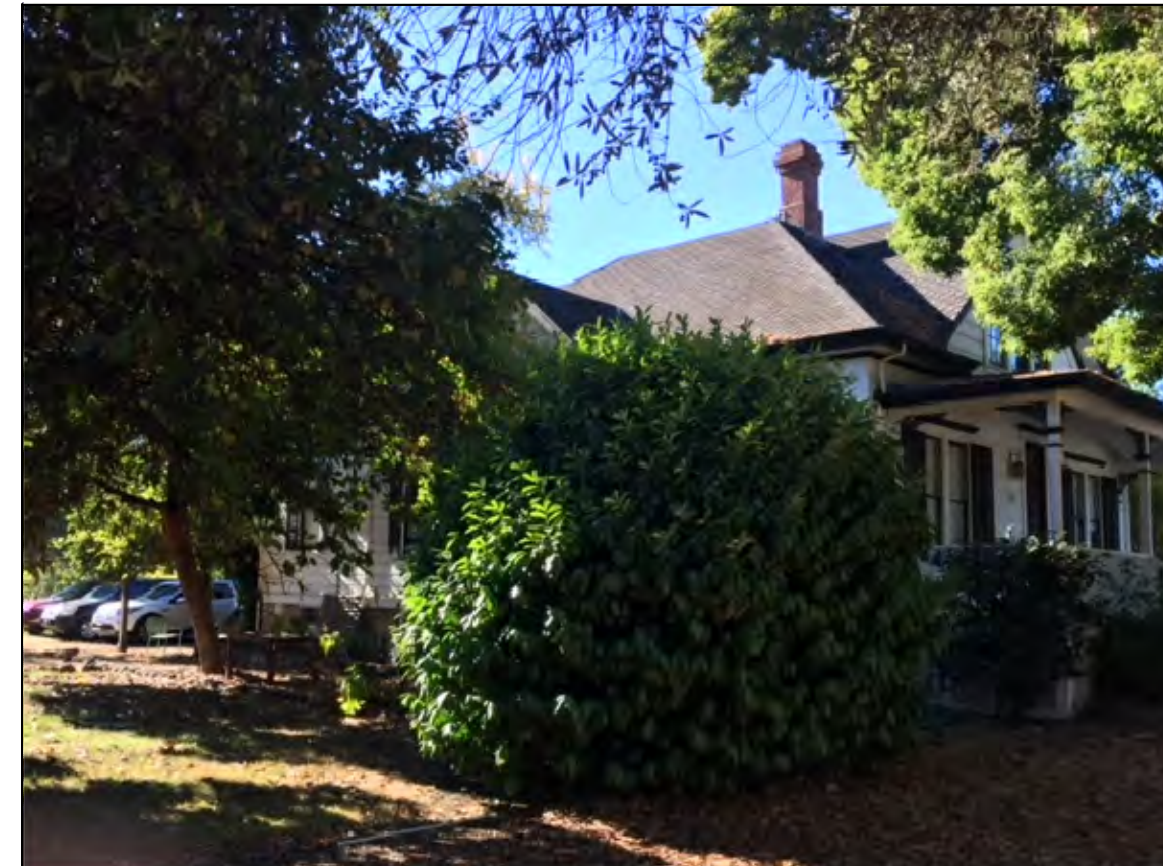
VIEW OF NE CORNER OF BUILDING
