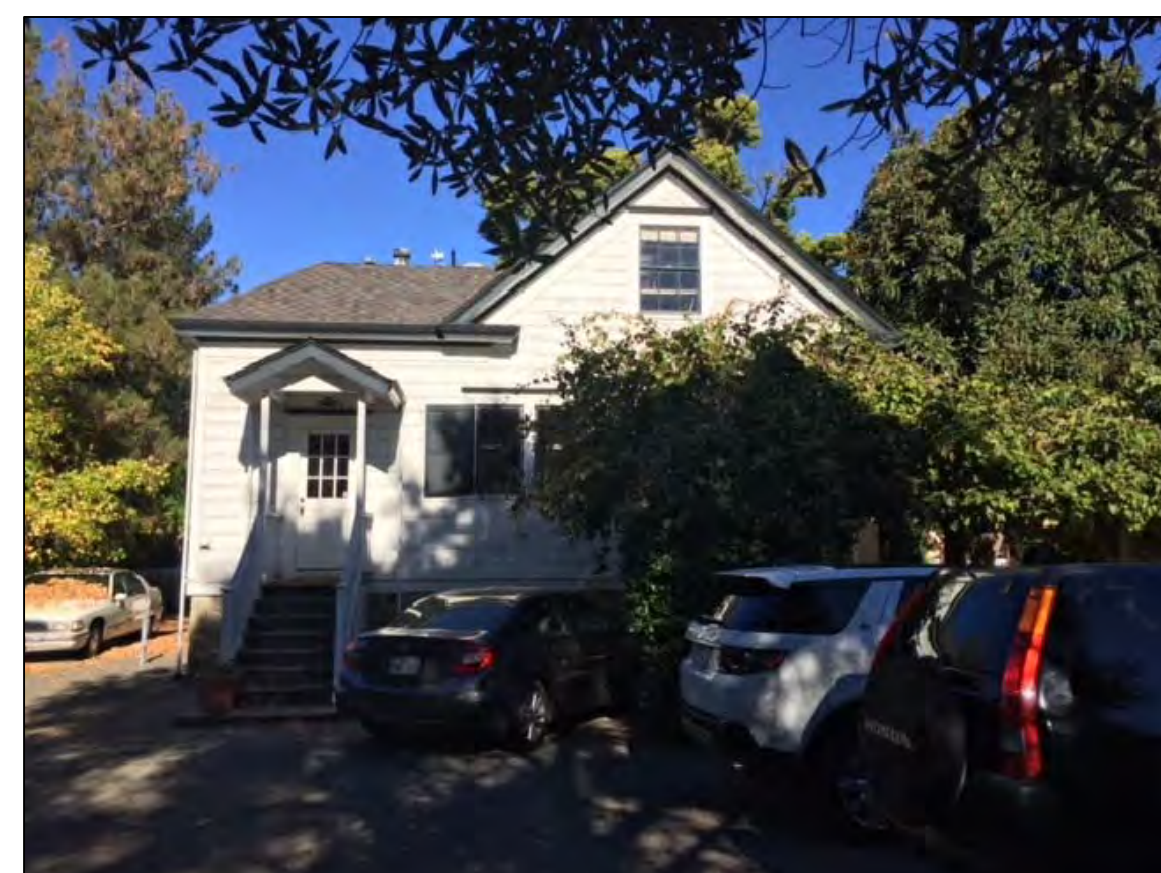
VIEW OF SOUTH SIDE OF BUILDING (REAR)
