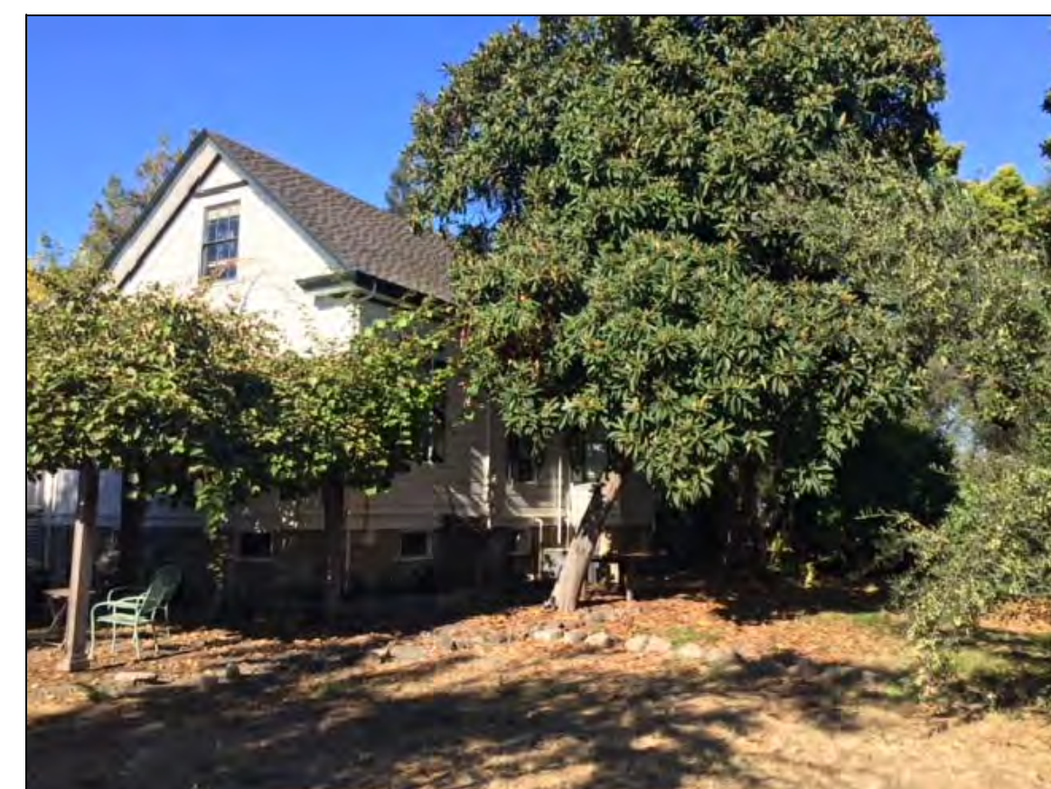
VIEW OF SE SIDE OF BUILDING
