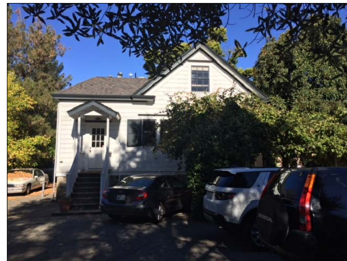
VIEW OF SOUTH SIDE OF BUILDING (REAR)
