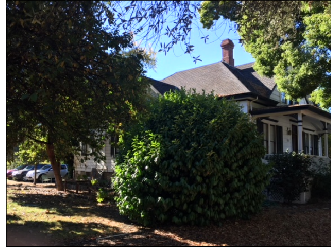
VIEW OF NE CORNER OF BUILDING
