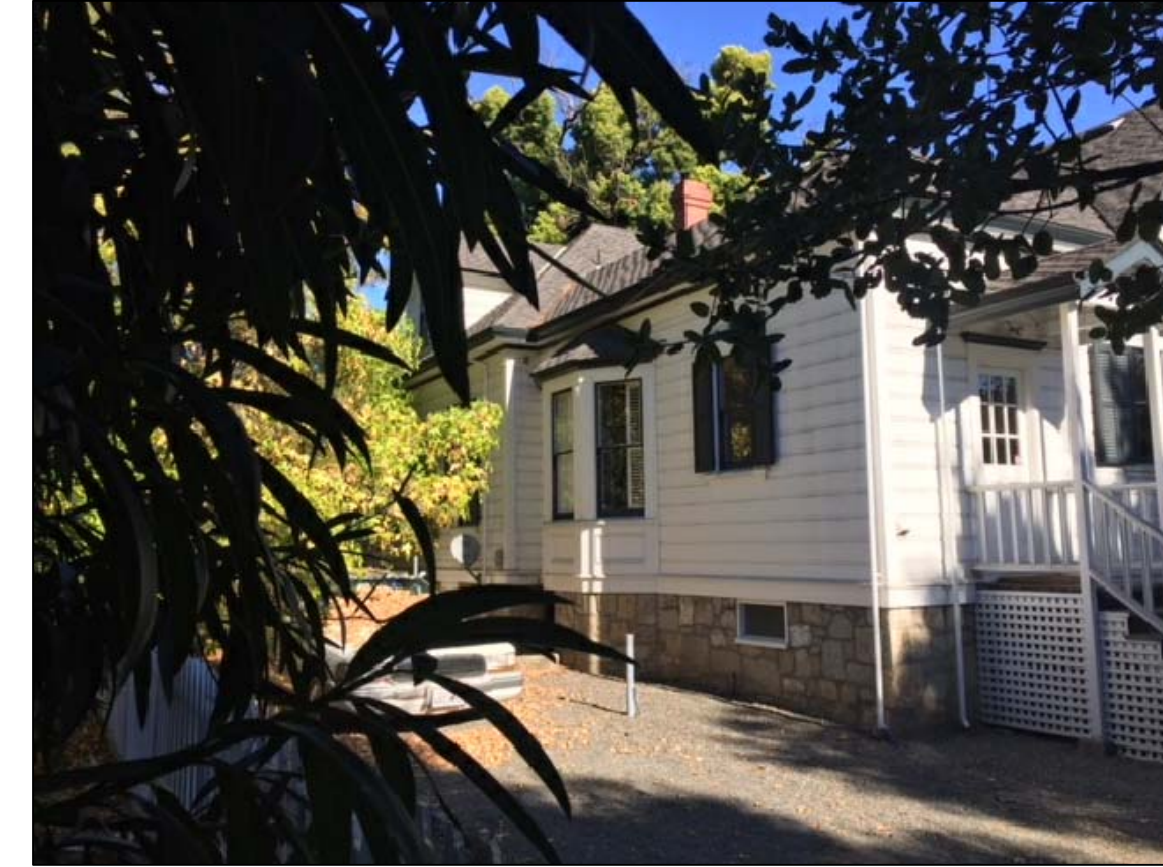
VIEW OF SW SIDE OF BUILDING
