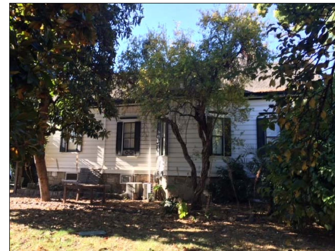
VIEW OF EAST SIDE OF BUILDING
