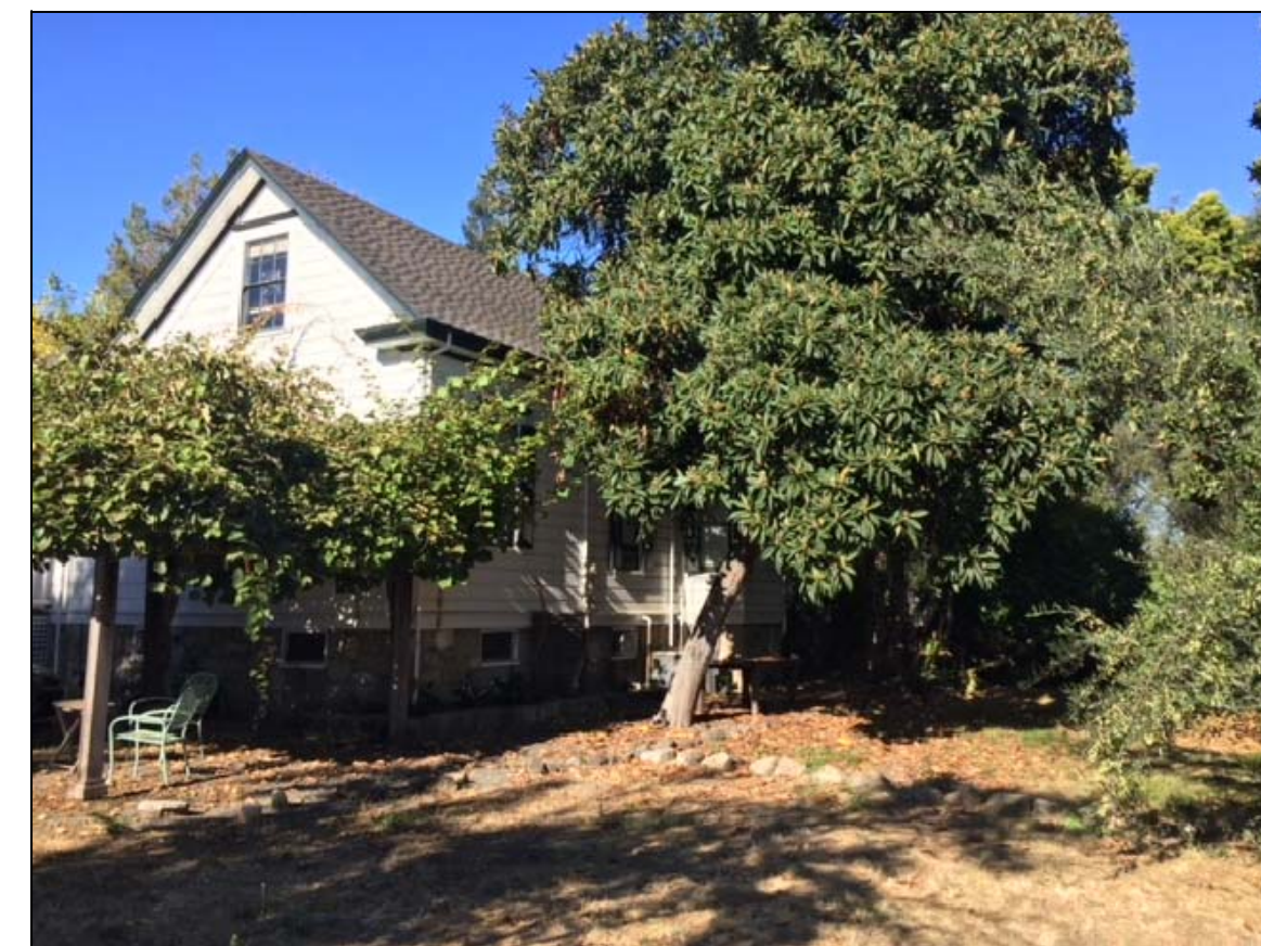
VIEW OF SE SIDE OF BUILDING
