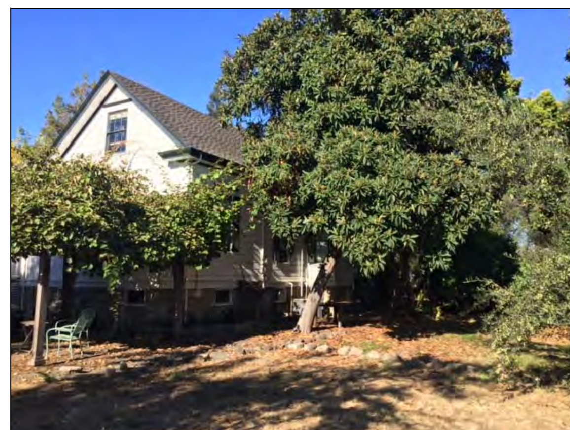
VIEW OF SE SIDE OF BUILDING
