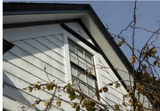
Figure 21: Divided-lite, single-hung, gable end window at rear façade. Looking north.
