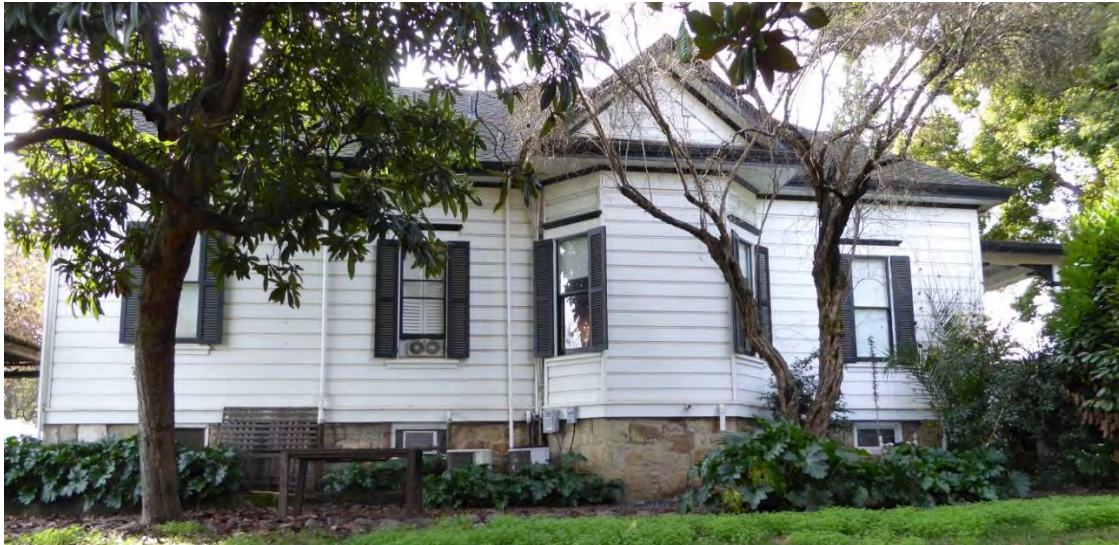
Figure 14: Northeast façade viewed from east side yard of subject property. Looking southwest.
