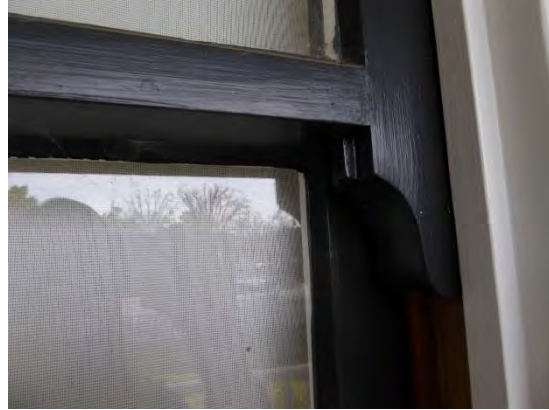
Figure 10: Detail of wood-sash window and ogee lug. Looking south.
