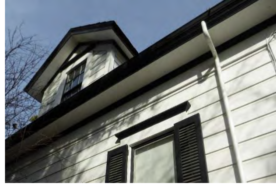
Figure 27: Dormer window above southwest façade. Looking north.
