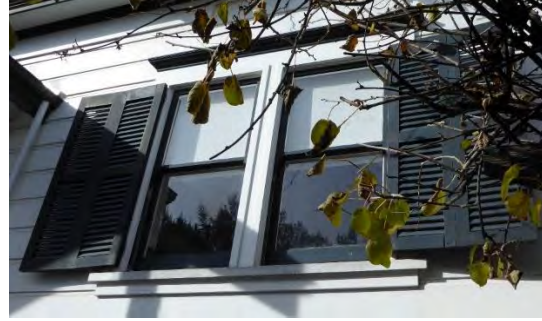
Figure 20: Paired standard windows to immediate east of rear entrance. Looking northwest.
