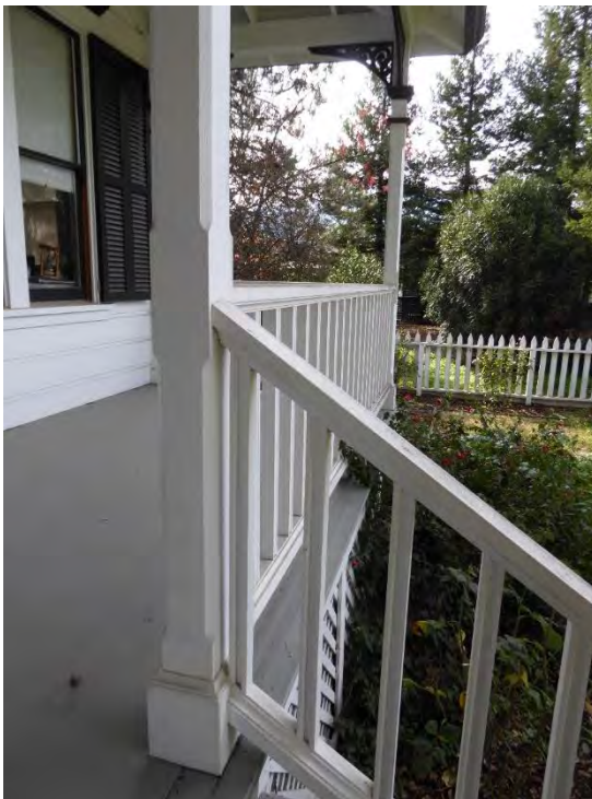
Figure 7: Railing, chamfered column, and balustrade along front porch. Looking southwest.
