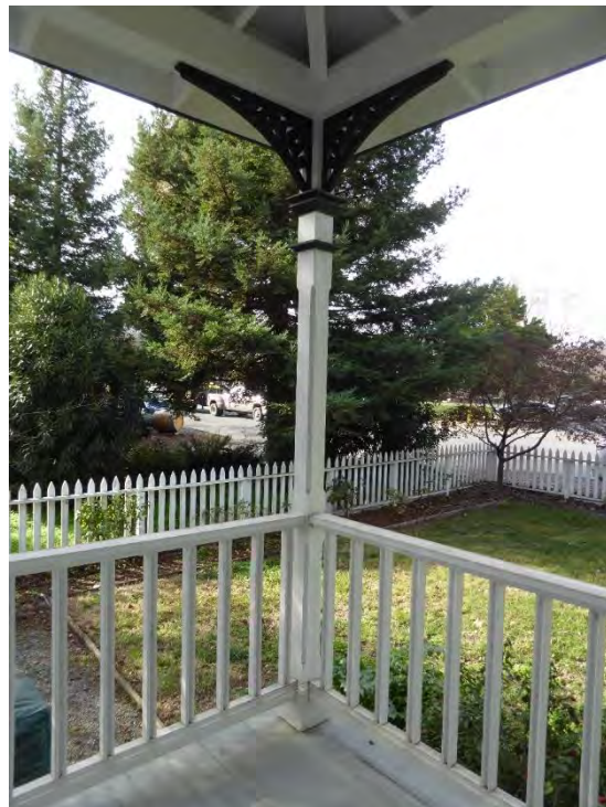
Figure 8: Column and non-original wood brackets at northwest corner of porch. Looking west.
