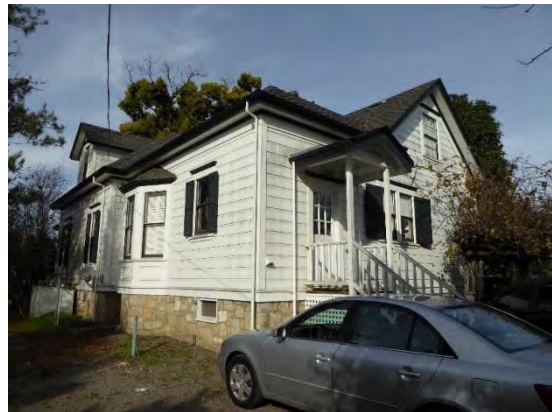
Figure 25: South end of southwest façade. Looking north.
