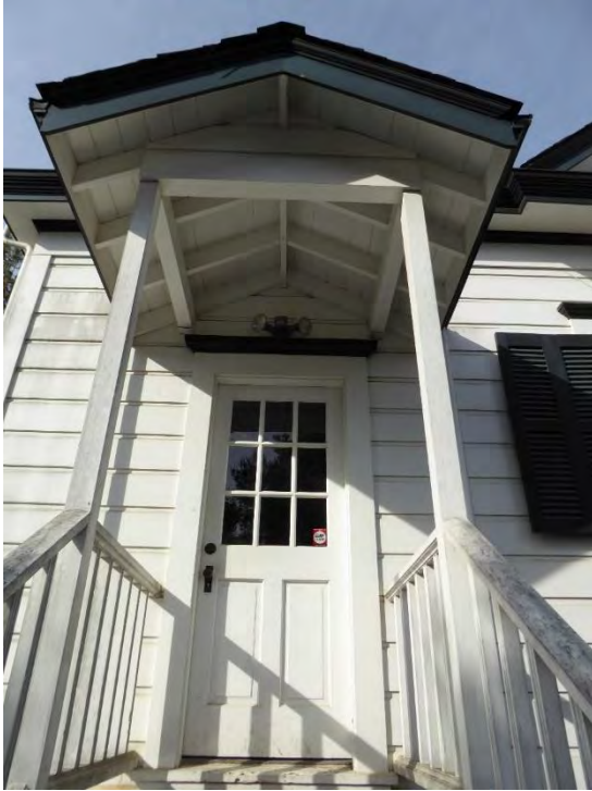
Figure 19: Covered stair landing at rear entrance. Looking northwest.
