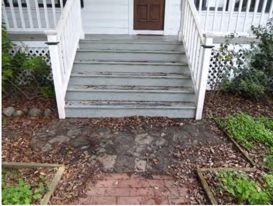
Figure 5: Wood steps with wood railing leading to porch. Looking southeast.
