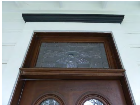
Figure 12: Transom with art glass above main entry door. Looking southeast.
