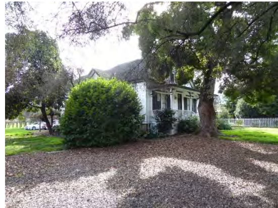
Figure 31: Subject building viewed from north corner of subject property. Looking south.
