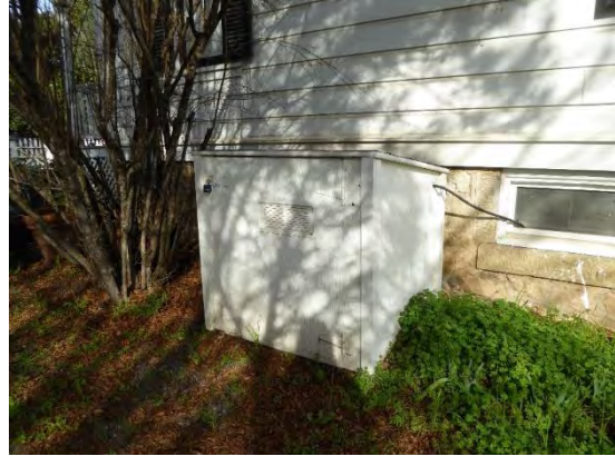
Figure 23: Utility box adjacent to partially raised basement at southwest façade. Looking north.
