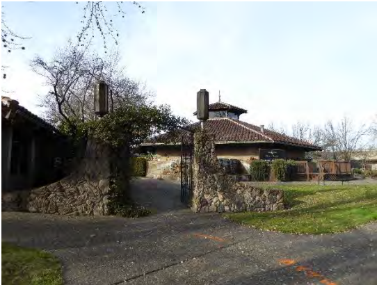
Figure 38: Entrance to Beaulieu Vineyards complex to along northwest side of Rutherford Road, to north of subject building.
