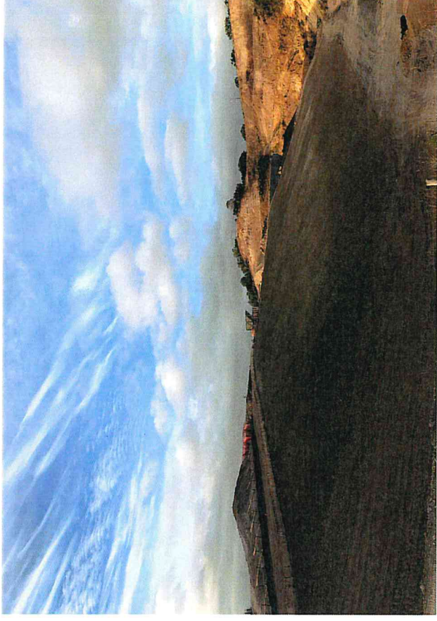
15k Yds soil cap and Hydroseed
