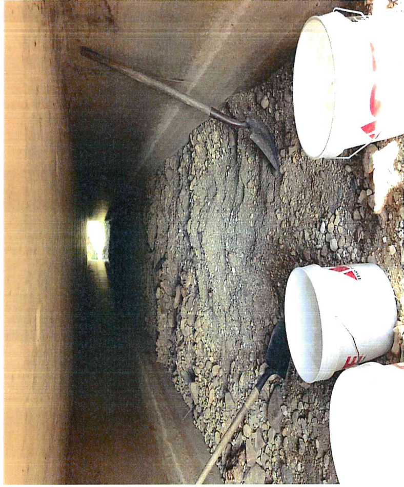
Culvert Sediment
