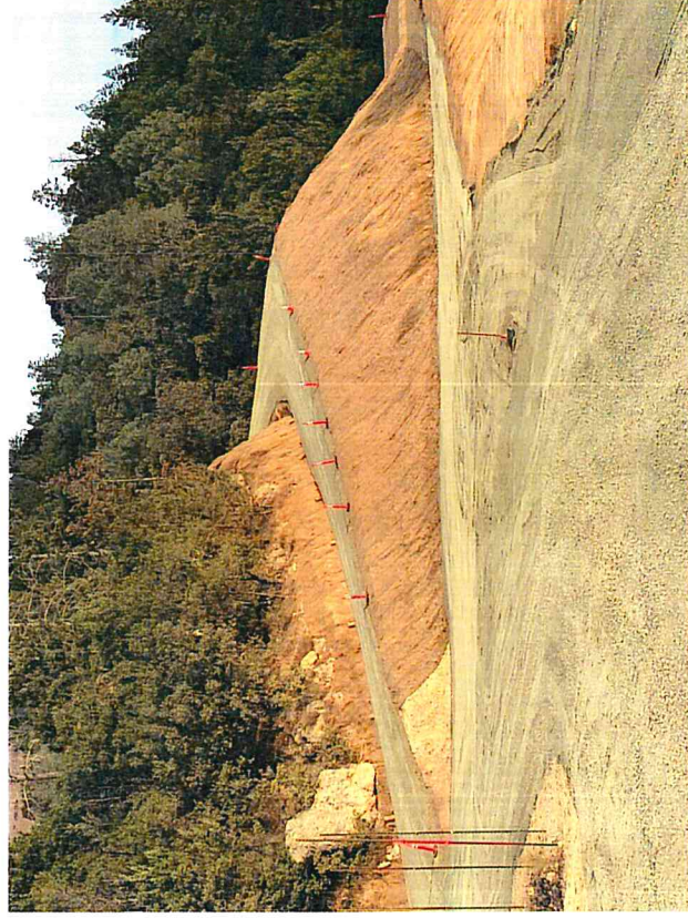
BMPs: Geotextile and Base Rock
