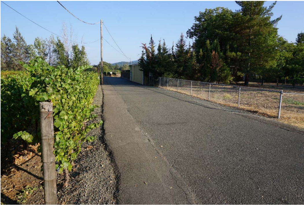
Sta 0+50, Looking from Tubbs Lane
