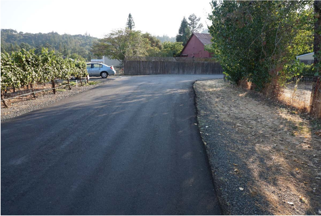
Sta 2+50, looking up station
