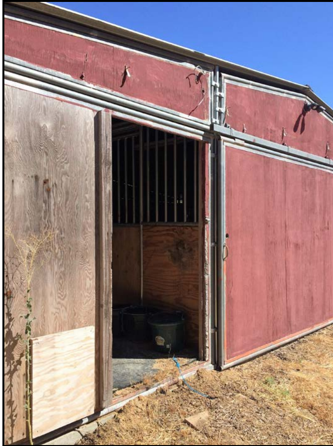
Photo 7: Onsite Barn/Storage Structure
