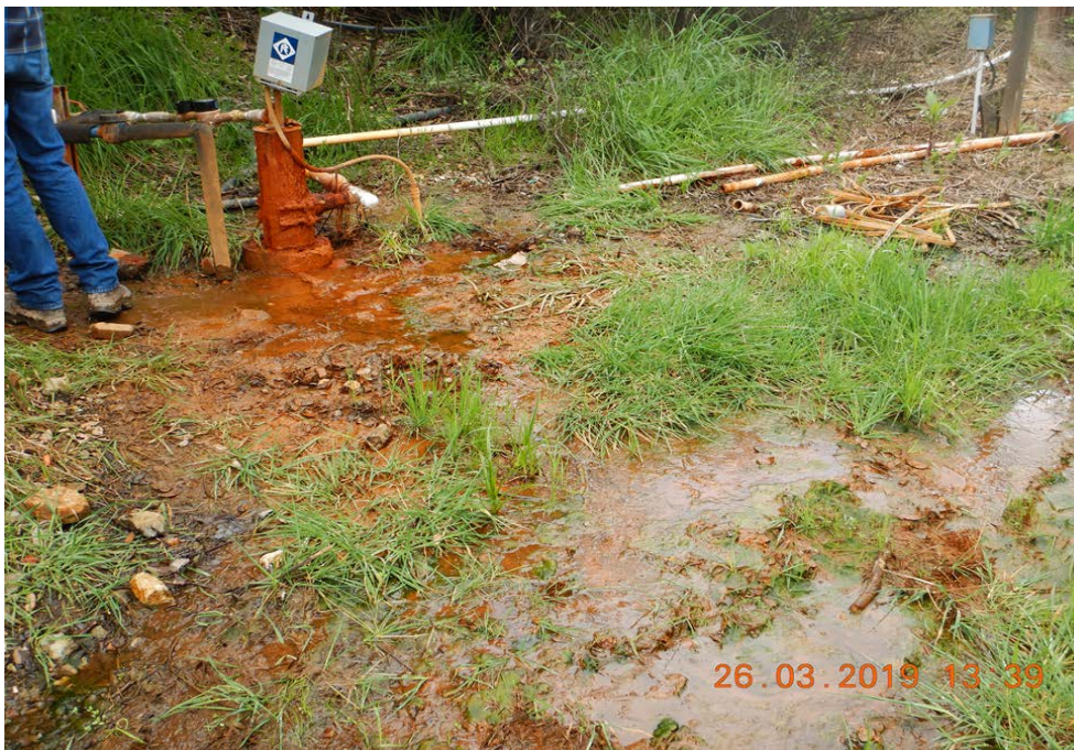
Photo 535- ponded leachate around the rusted LEW2 wellhead, looking northwest.
