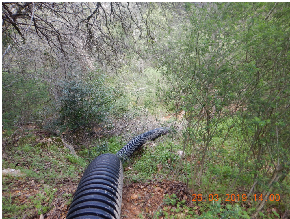
Photo 575- pipeline from the landfill into the creek, looking east.
