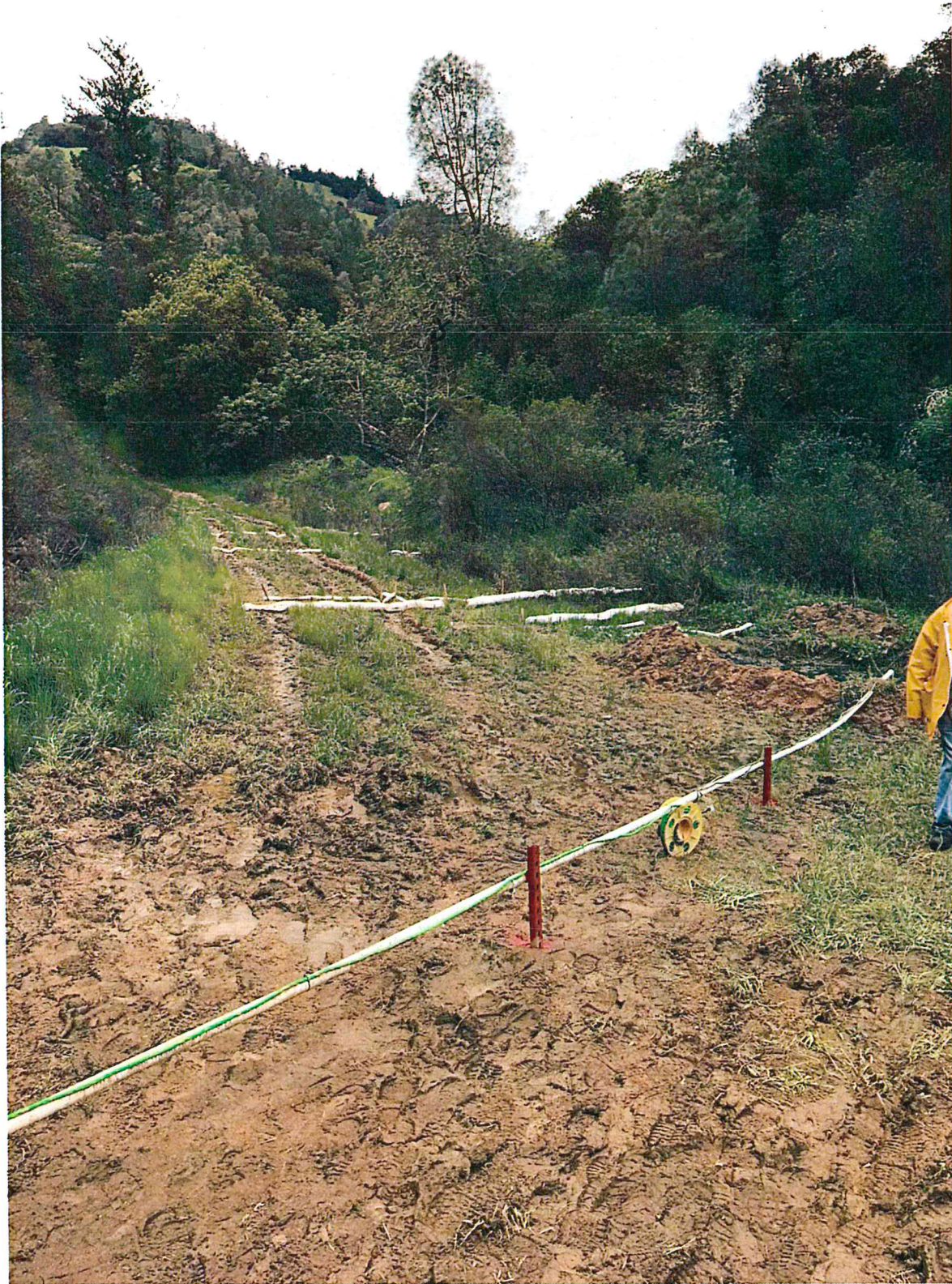
Exhibit 2 - flow around basin at creek #1 4-2-19
