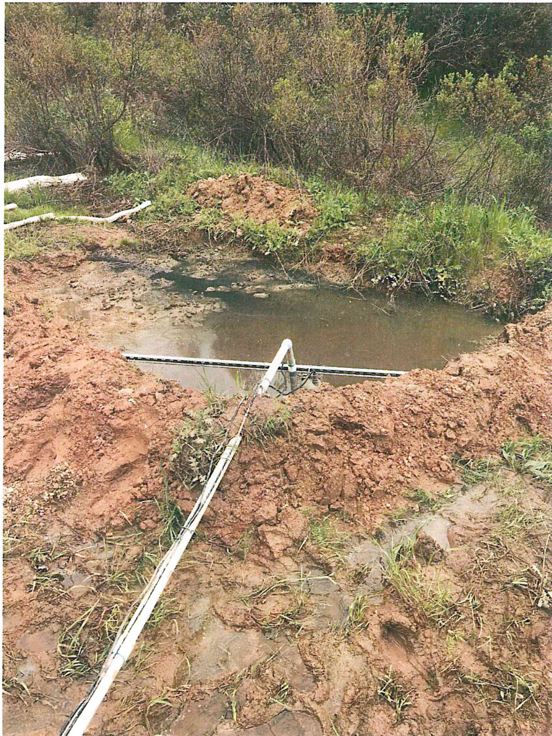
Exhibit 3 - flow around basin at creek #2 4-2-19
