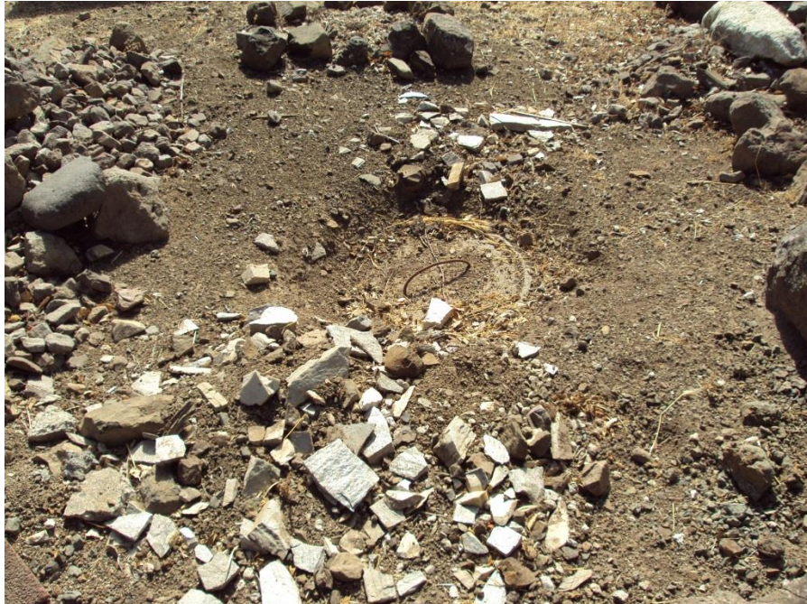
Photograph 22: Easterly view of septic tank risers. June 23, 2014
