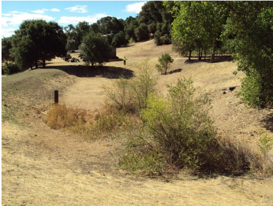
Photograph 35: Southeasterly view of stormwater detention/infiltration basin and riser. June 23, 2014
