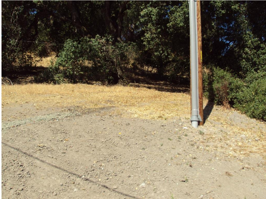
Photograph 44: Westerly view of recently installed power pole behind residence. June 23, 2014
