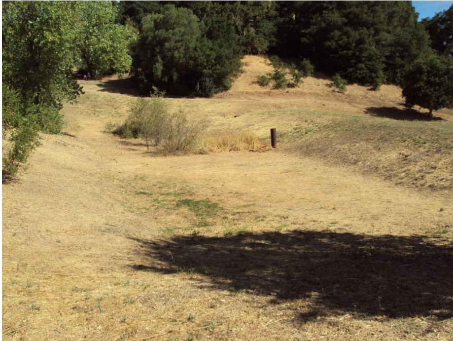
Photograph 33: Northwesterly view of stormwater detention/infiltration basin and riser. June 23, 2014
