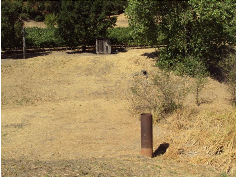
Photograph 34: Southwesterly view of stormwater detention/infiltration basin, well pump house and riser. June 23, 2014
