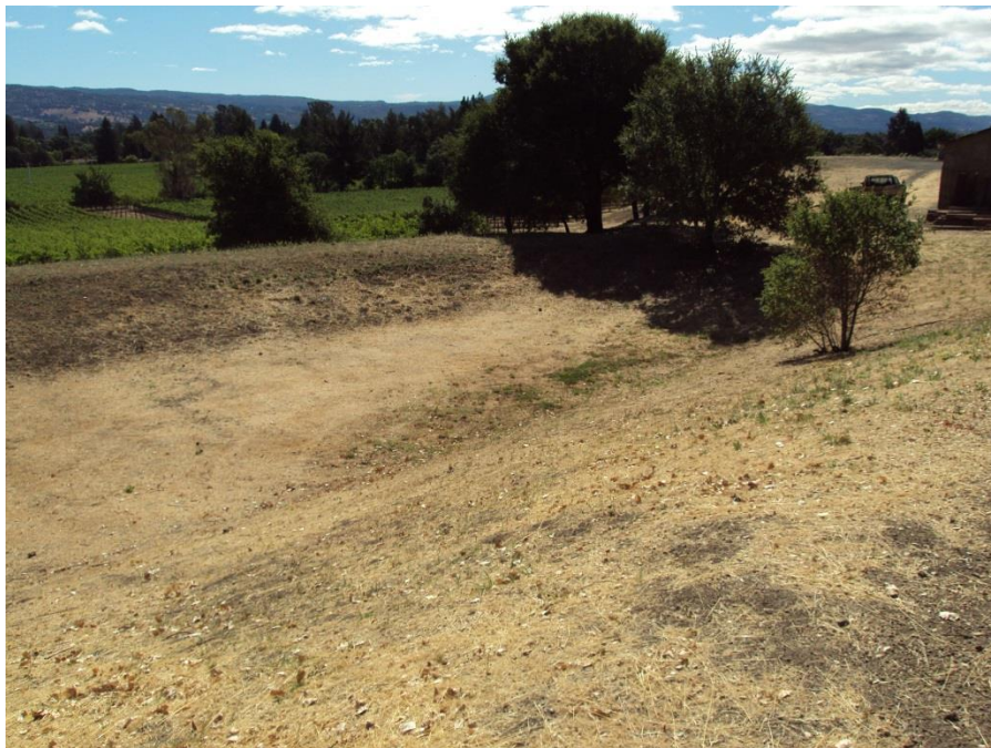
Photograph 36: Easterly view of stormwater detention/infiltration basin, vineyard and barn. June 23, 2014
