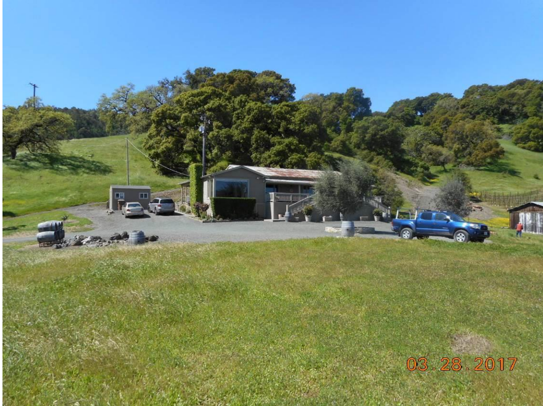
Photo 1. View of the area proposed for offices, guest parking, and tasting room.
