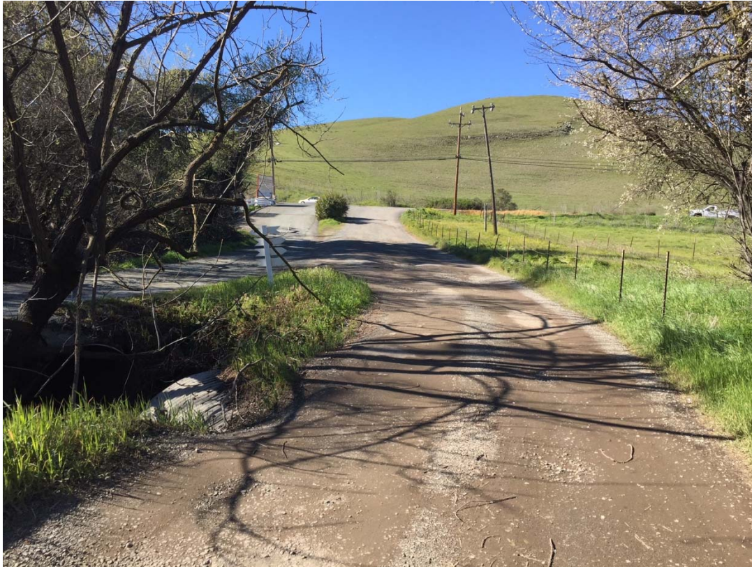
Photo 1. Access road and culvert facing east. March 2018.
