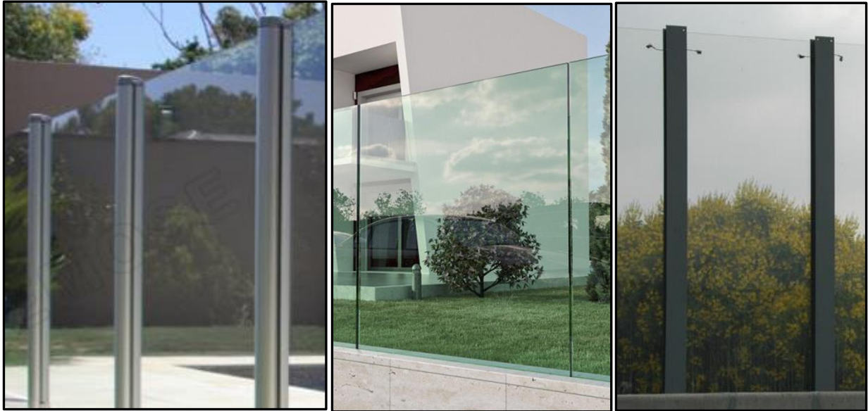
Figure 6: Examples Clear Acoustical Barrier Panel Installations
