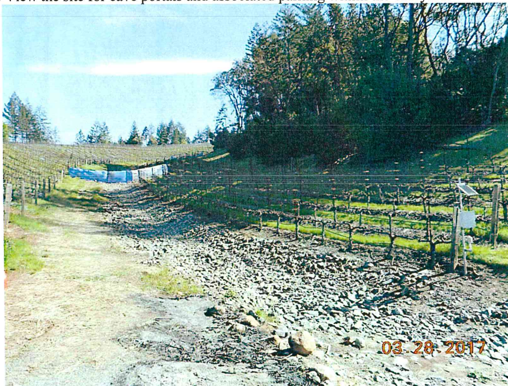
Photo 5. View of the access road that will serve the hospitality building and winery cave portals.
