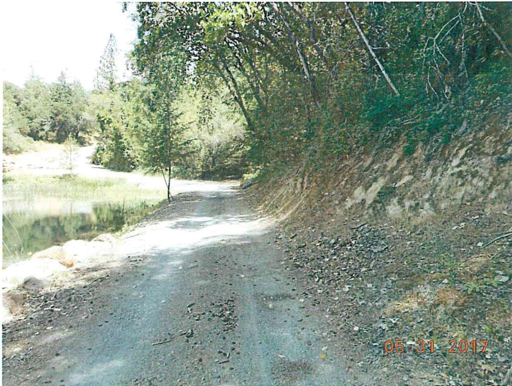
Photograph 1. Project site illustrating where the entrance road will be widened. Napa False Indigo is growing along the upper bank of the area that will be graded to meet access road standards.
