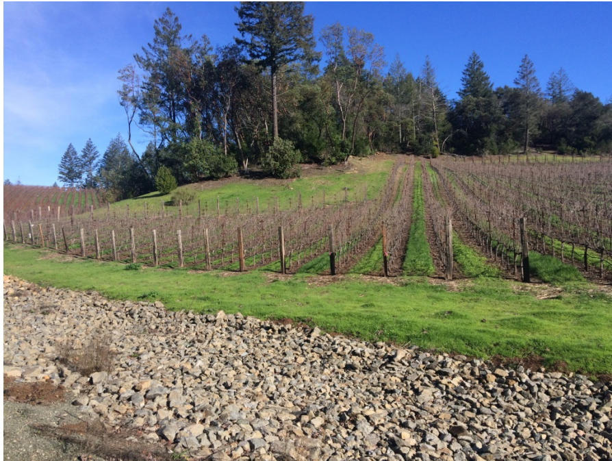
Photograph 7: Northeasterly panoramic view of rock lined swale, gravel access road and vineyard. January 26, 2016
