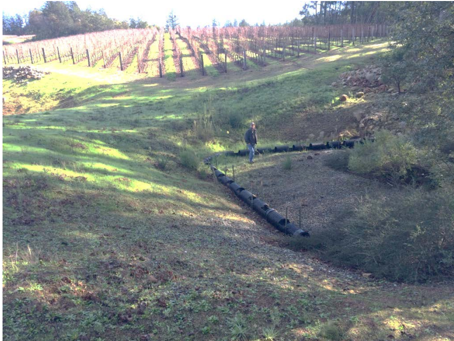
Photograph 33: Southeasterly view of a drainage course, vineyard, gravel access road and outlet Tee spreader. January 26, 2016
