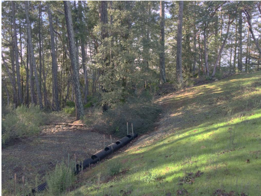
Photograph 39: Southwesterly view of forested area and basin outlet Tee spreader. January 26, 2016
