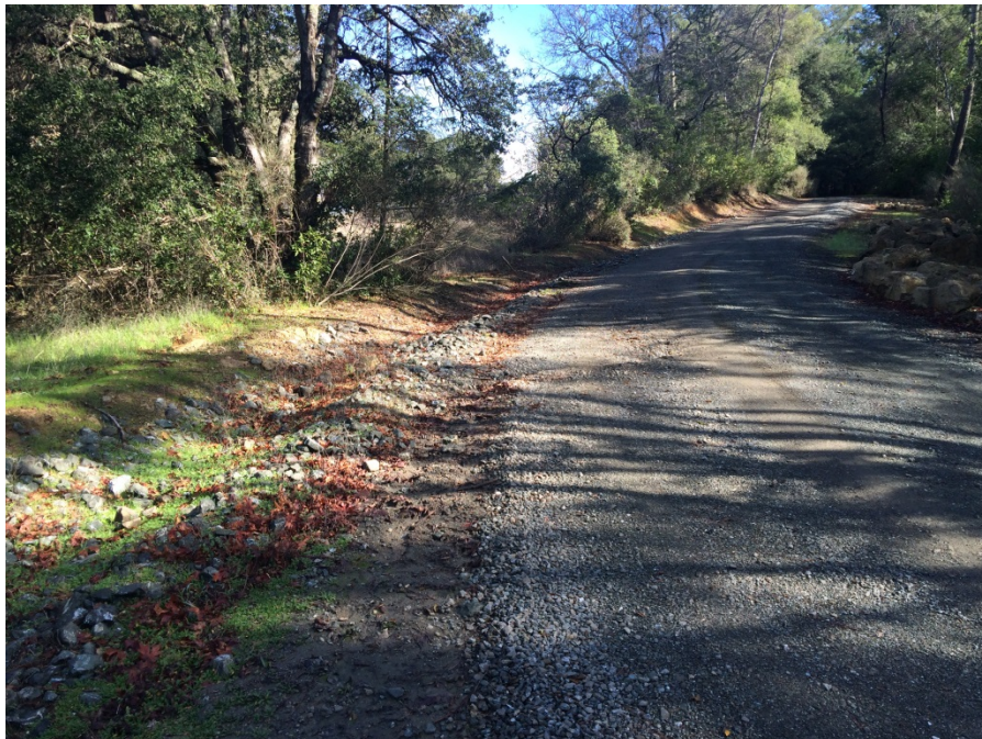
Photograph 104: Easterly panoramic view of gravel access road, drainage course and vegetation.
