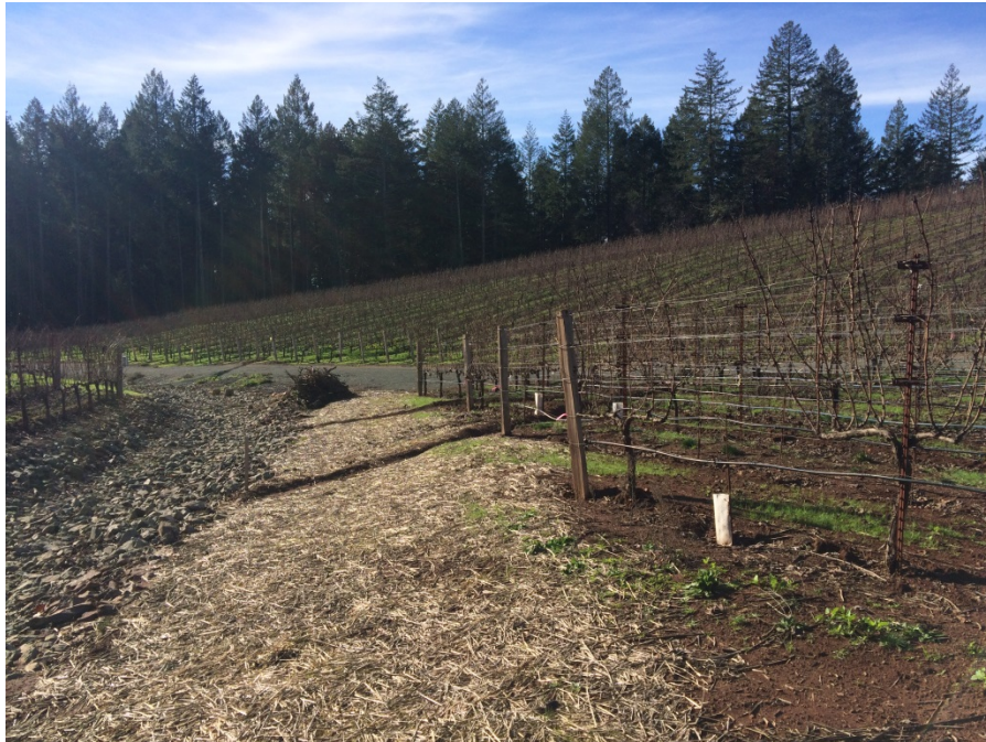
Photograph 23: South southwesterly panoramic view of rock lined swale, gravel access road and vineyard. January 26, 2016
