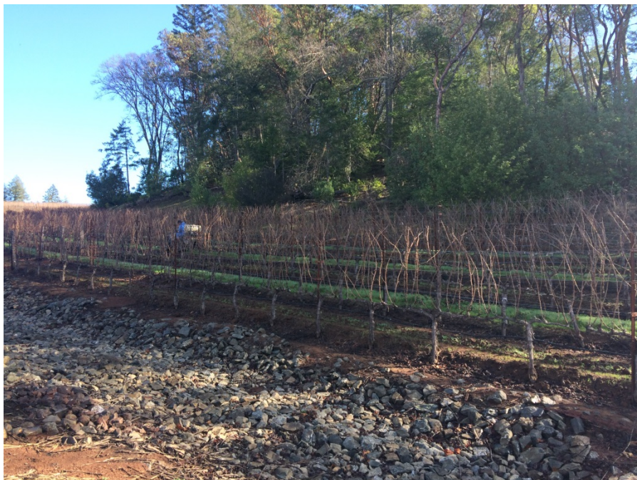
Photograph 20: East northeasterly panoramic view of rock lined swale, gravel access road and vineyard. January 26, 2016
