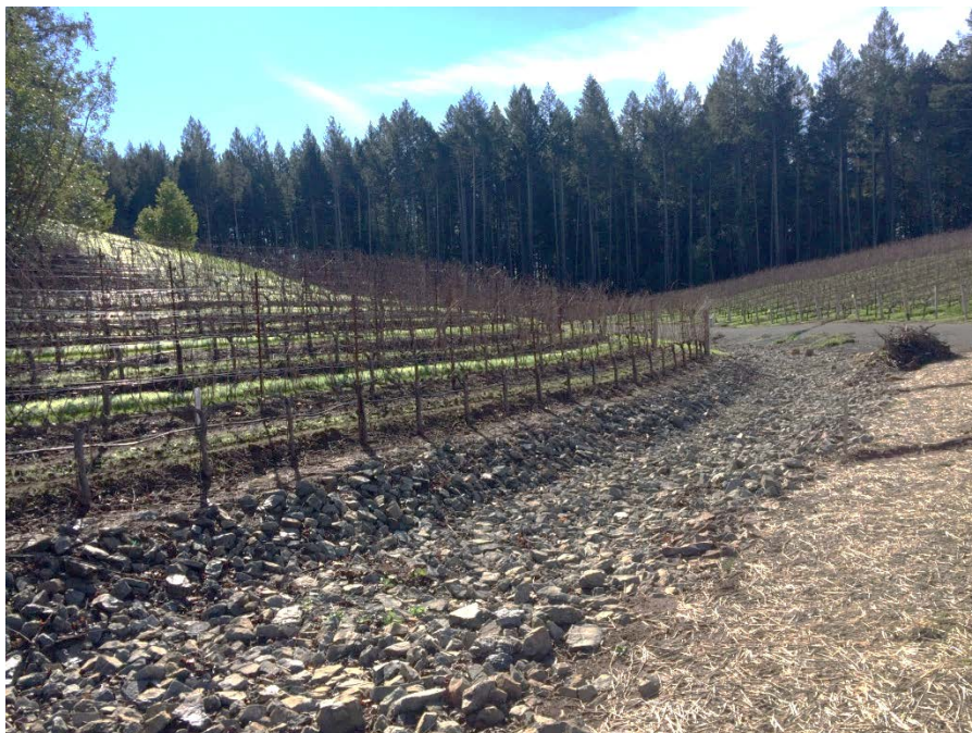
Photograph 22: South southeasterly panoramic view of rock lined swale, gravel access road and vineyard. January 26, 2016
