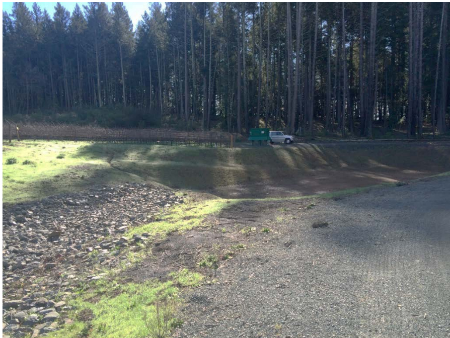
Photograph 10: South southeasterly panoramic view of gravel access road, rock lined swale and basin. January 26, 2016
