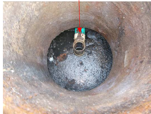
T's are in place.
