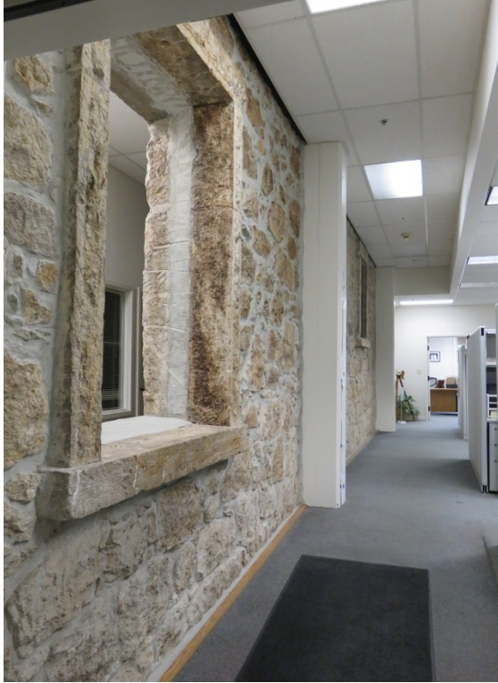
1930 addition office areas (right) and former exterior wall c.1885 winery addition (left), note sandblasted stone walls and window removal
