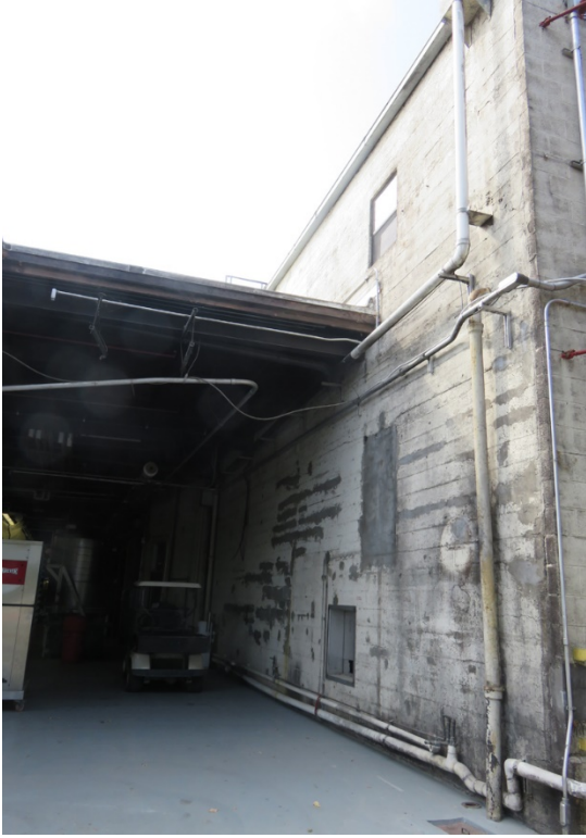
View south down rear elevation of 1941 addition
