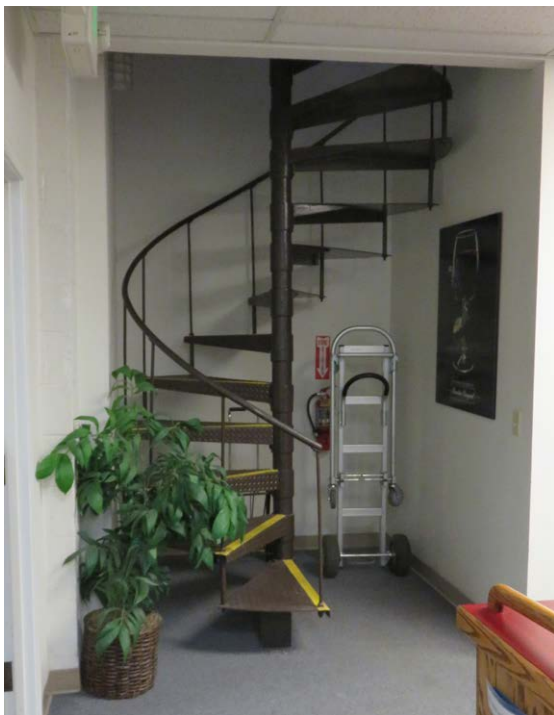
Spiral staircase, 1941 addition
