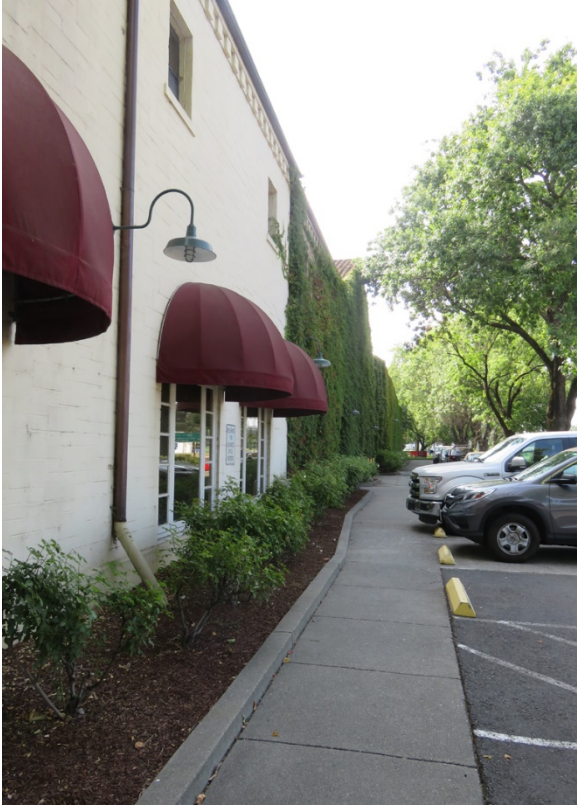
View south along front (west) elevation, from office entrance
