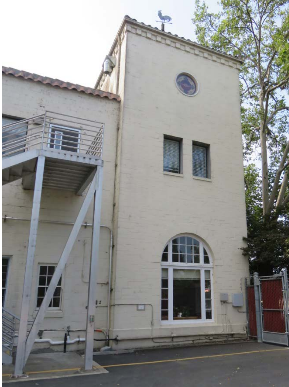
North elevation, tower at northwest corner
