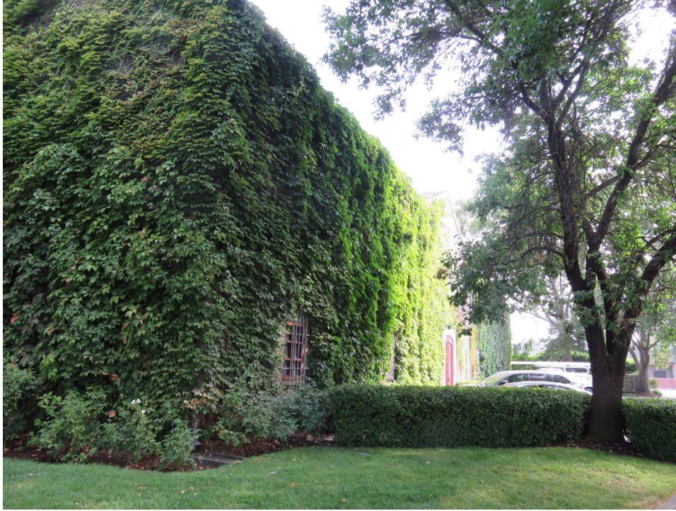
View east along south elevation, 1974 addition
