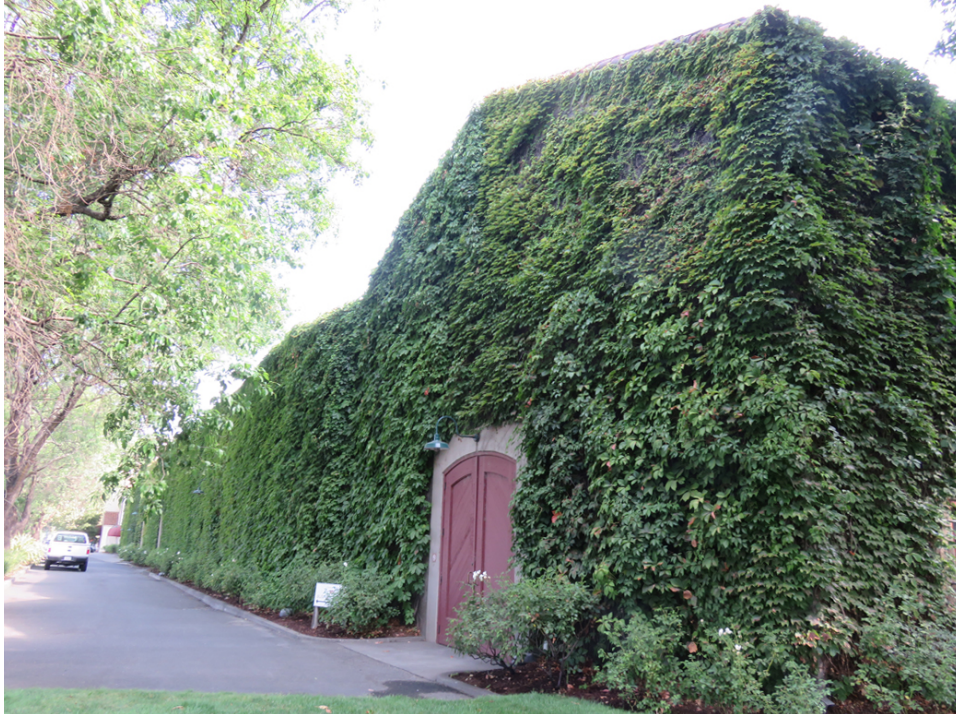
View north along front (west) elevation from southwest corner
