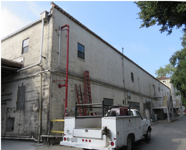
View west down north elevation of 1941 addition
