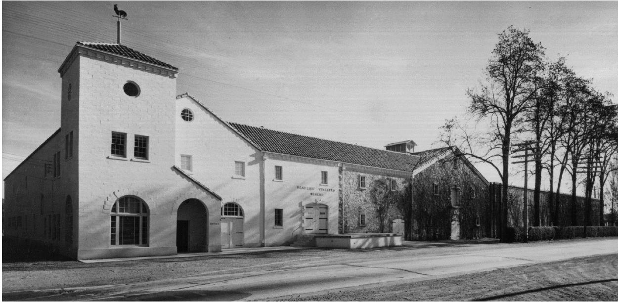
Following completion of concrete masonry unit addition in 1941 (Photo: Napa County Historical Society)
