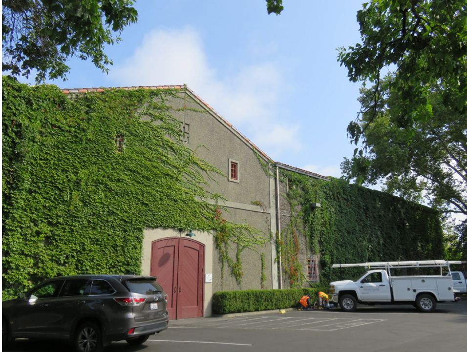
South elevation of 1974 addition
