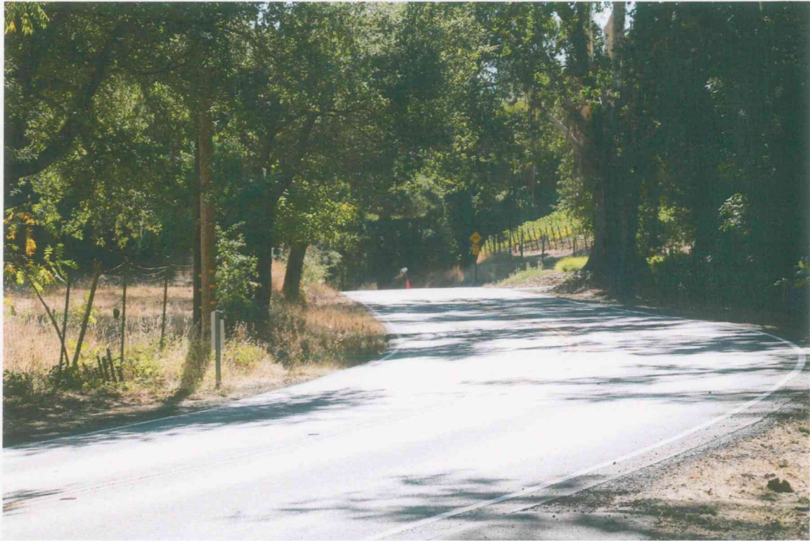
Photo 1 - Looking south from centerline of driveway - cone & flag placed 500' away
