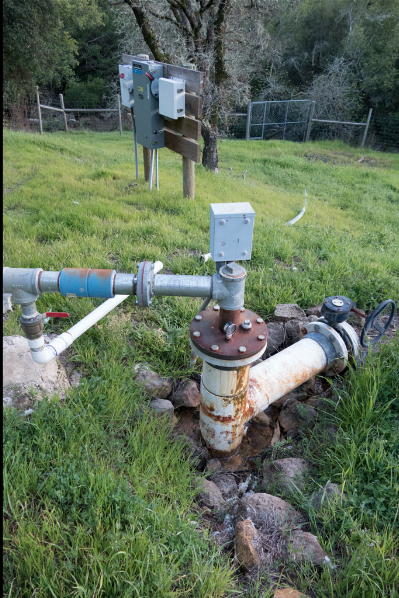
Well casing failure?
